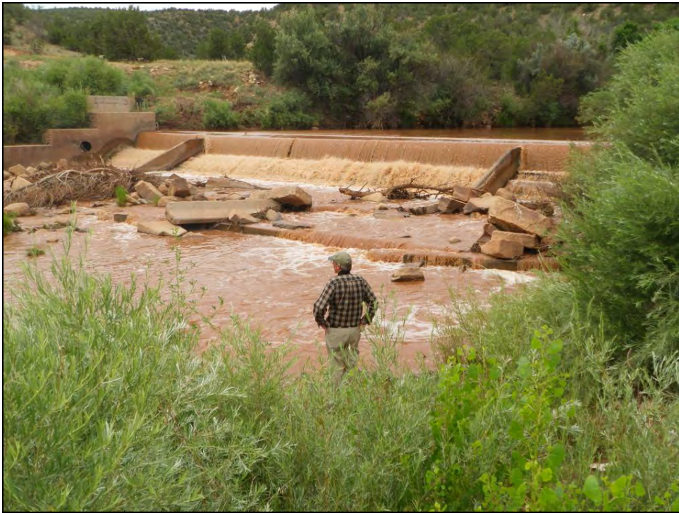
Photograph No. 36: Overview of the Villanueva Diversion Structure, from downstream on the north bank. July 15, 2014.
