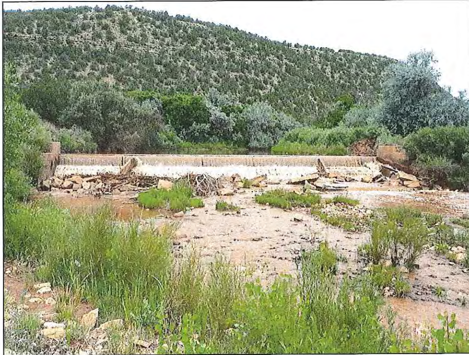
Photograph No. 6: Overview of the Villanueva Diversion Structure, from downstream. July 15, 2014.
