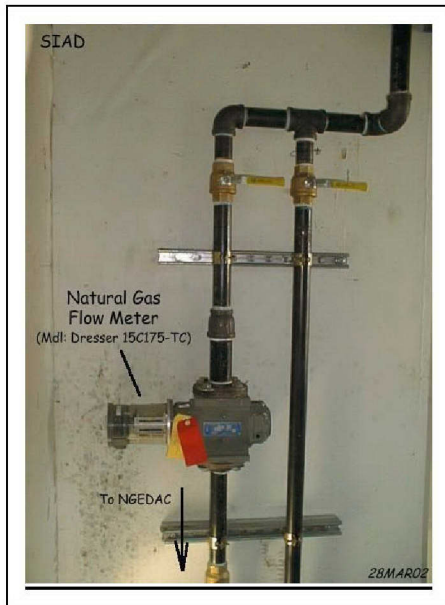
Figure 12. Natural gas flow meter.
