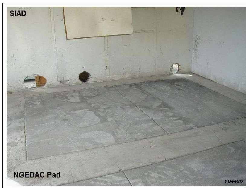
Figure 7. Reinforced compressor pads.
