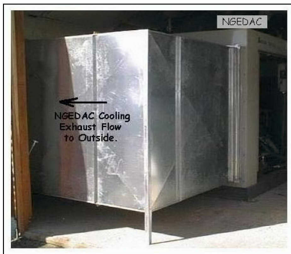
Figure 8. NGEDAC cooling exhaust.
