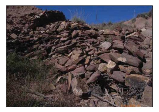
Figure 4.9. Remnants of masonry armoring river bank, facing northwest (uphill) toward earthen berm.
