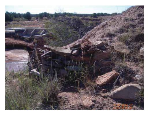
Figure 4.7. Northern end of eastern retaining wall, arcing inward toward the earthen berm.
