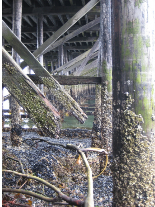
Figure D-5. View underneath causeway
