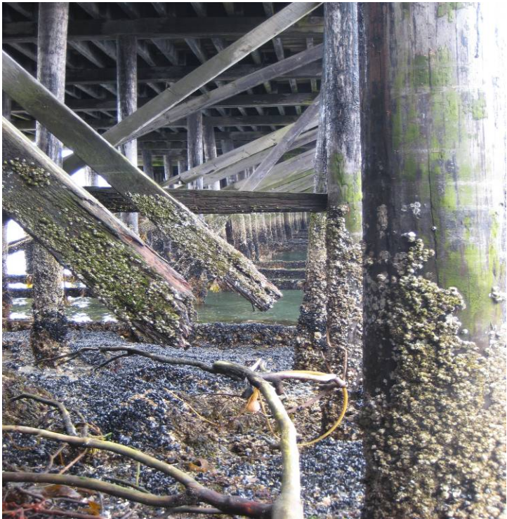
Figure 9. Underside of Dock
