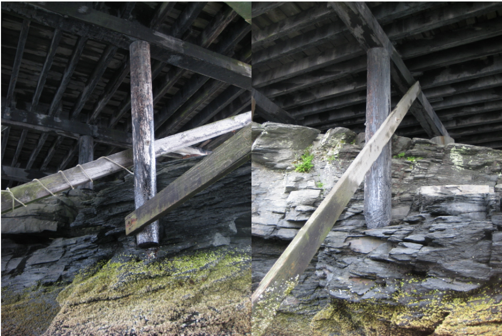
Figure D-3. Unbraced piles on bedrock
