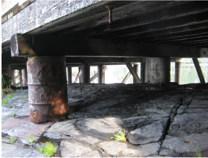
Figure D-9. Unbraced concrete barrel supports atop bedrock under causeway
