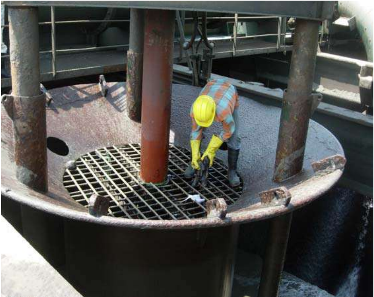
Figure 2-4. Photo of Observer Checking the Overflow Screen (Courtesy USACE ERDC)
