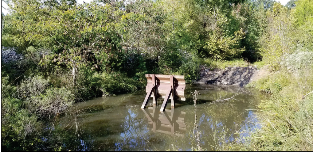
Figure 6. Campbell Creek grade control structure #1.
