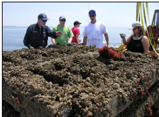
Figure 1. Subtidal Modular Concrete Oyster Reef, lower Rappahannock River, Virginia, heavily colonized by oysters and hooked mussels.
