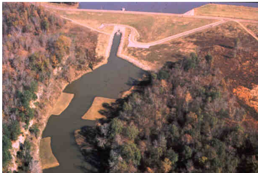
Figure 1. Gravel bar habitat in the upper end of an abandoned channel of the Tombigbee River, Mississippi, immediately after construction, 1985
