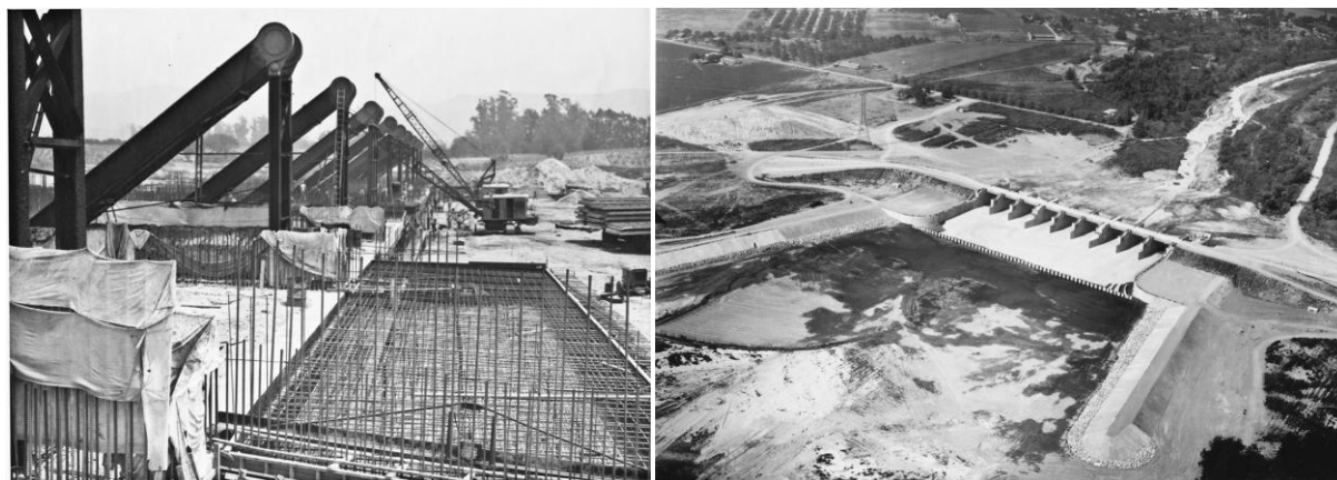
Construction of the Dam and Spillway
