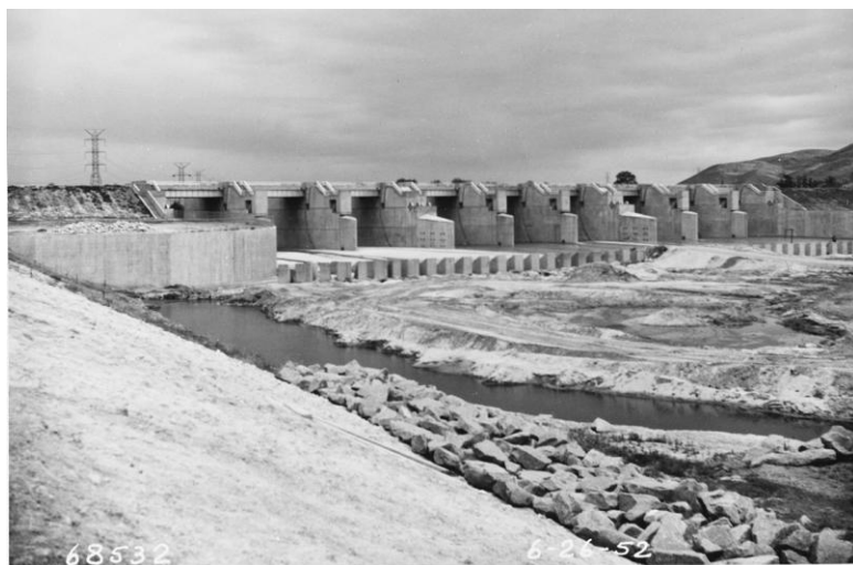
Whittier Narrows Spillway, 1952
