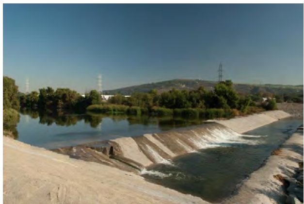
Drop Structure on San Gabriel River
