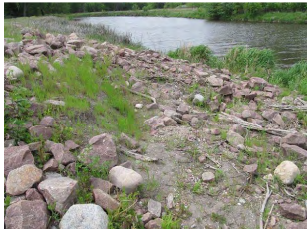
Figure 7. Chippewa River Diversion approach channel – west bank.
