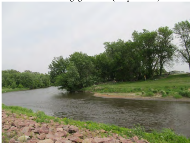
Figure 6. Chippewa River Diversion approach channel bank – upstream end (4 April 2012).
