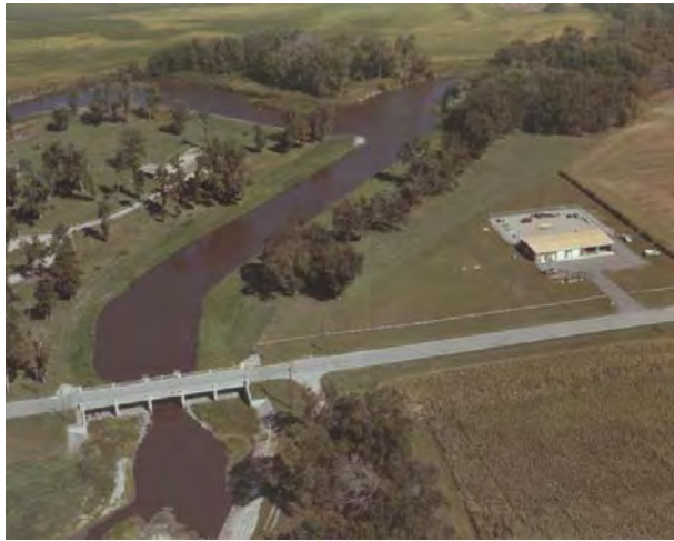
Figure 2. Chippewa River Diversion approach channel and control structure before erosion problems.
