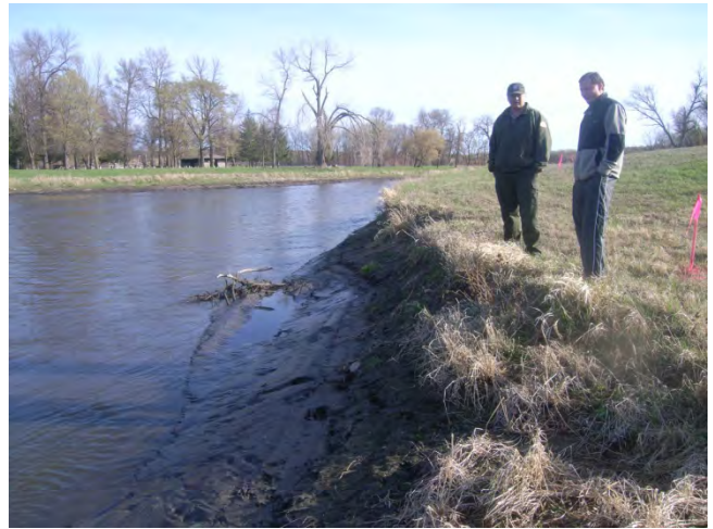
Figure 3. Chippewa River Diversion approach channel east bank - downstream reach (4 April 2012).
