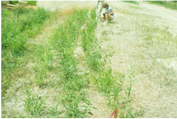
Figure 4. An establishing live stake area
