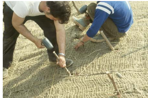
Figure 2. Installing a live stake
