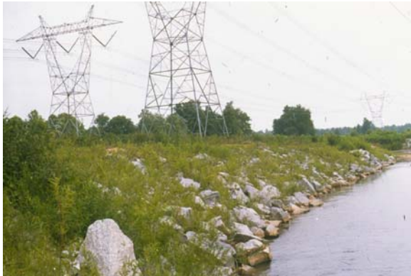
Figure 5. An establishing joint planting area
