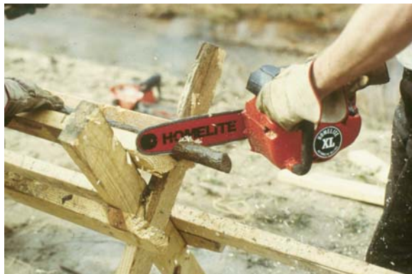
Figure 1. Fabricating a live stake or joint planting unit
