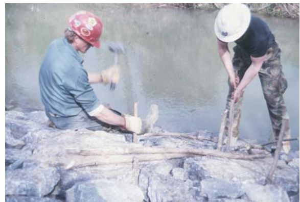
Figure 3. Installing a joint planting
