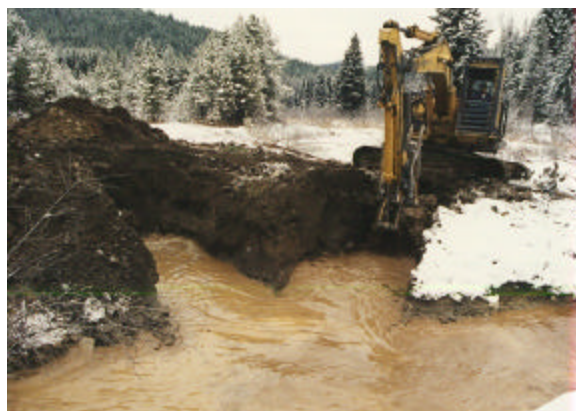
Figure 11. Trenches for rootwad bole and footer log
