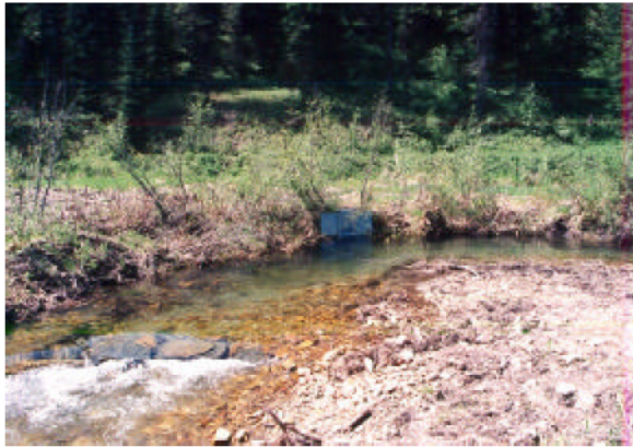
Figure 6. Use of rootwad composites with canal check and modified weir design.
