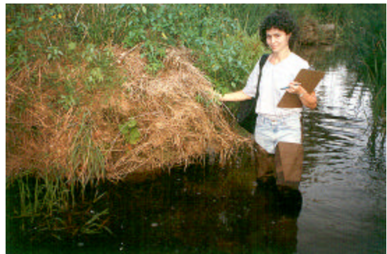
Figure 3. Rootwad composites can offer substantial habitat complexity. Prior to installation of rootwad composites, this streambank was raw and eroding
