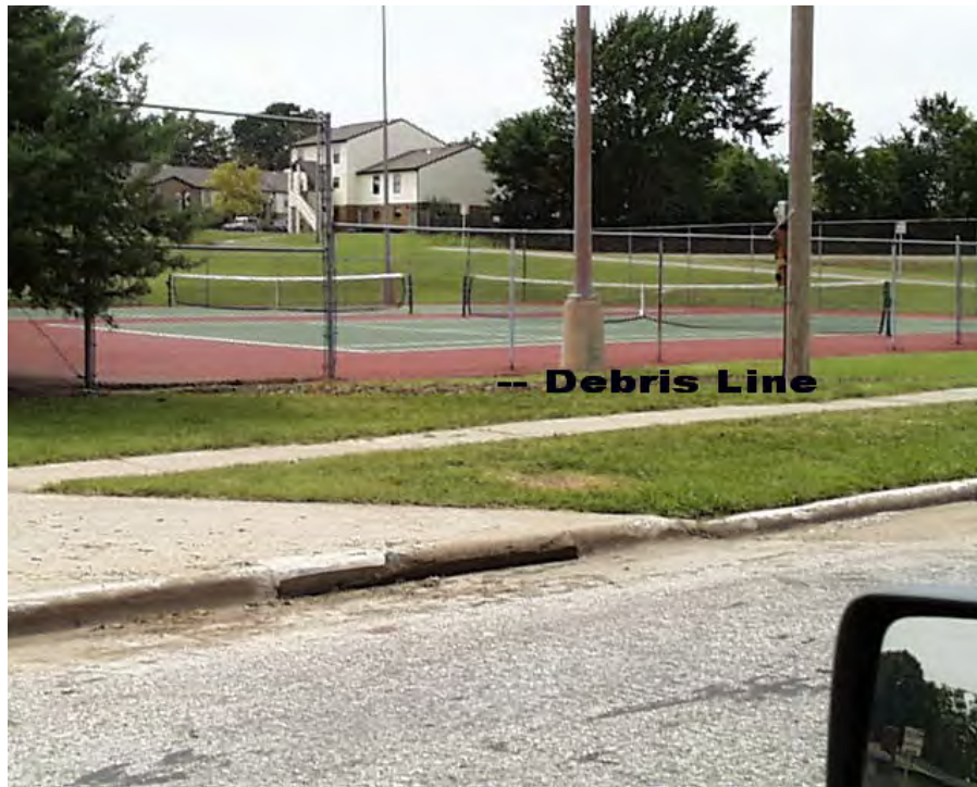
North Branch of Jordan Creek, on N Hampton Avenue crossing. (North Branch RS 3825). The debris line on the ground is estimated at elevation 1292+. This photo was taken after flood waters receded on July 12, 2000. See Appendix F for WSE comparison.
