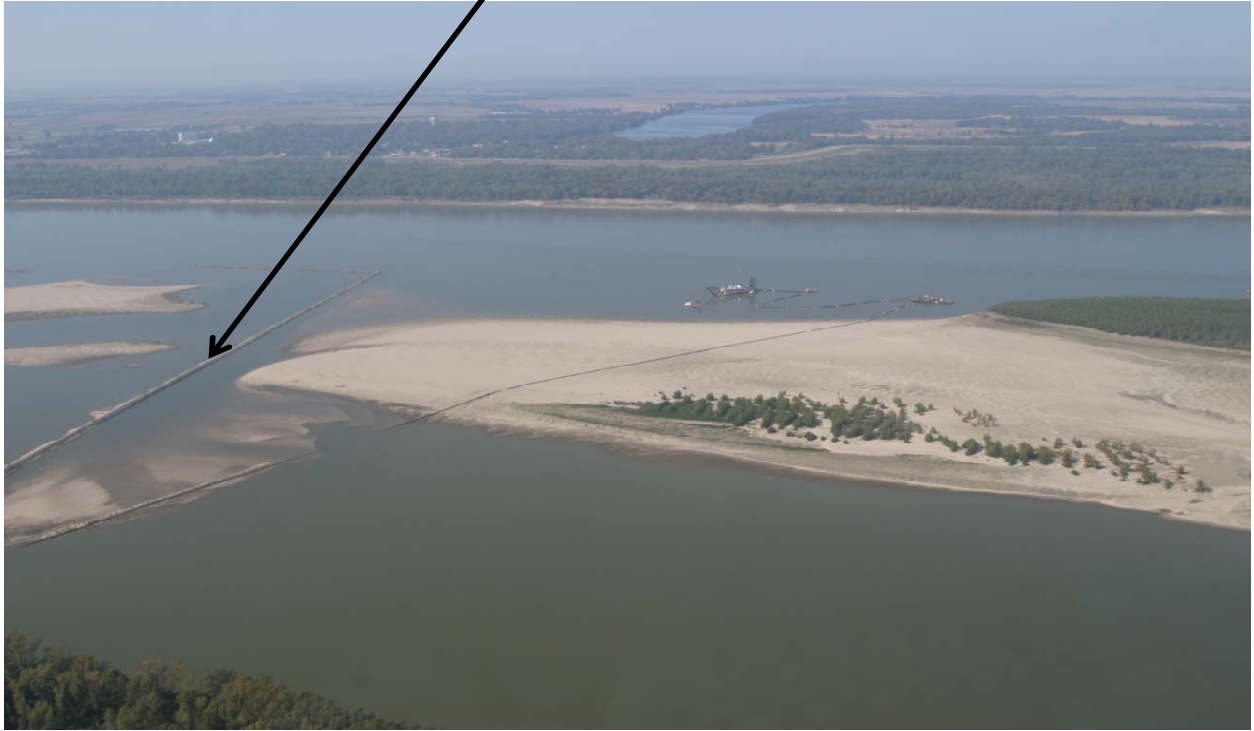
a. Closing dike at upstream reach of secondary channel.
