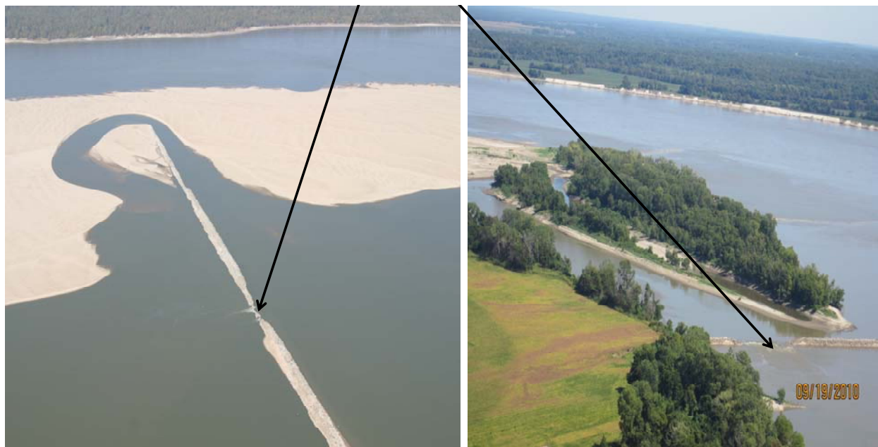
Figure 2. Notches through secondary channel dikes.
