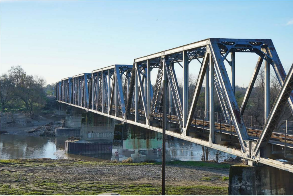
Photo 03: Railroad Bridge in phase 2A
