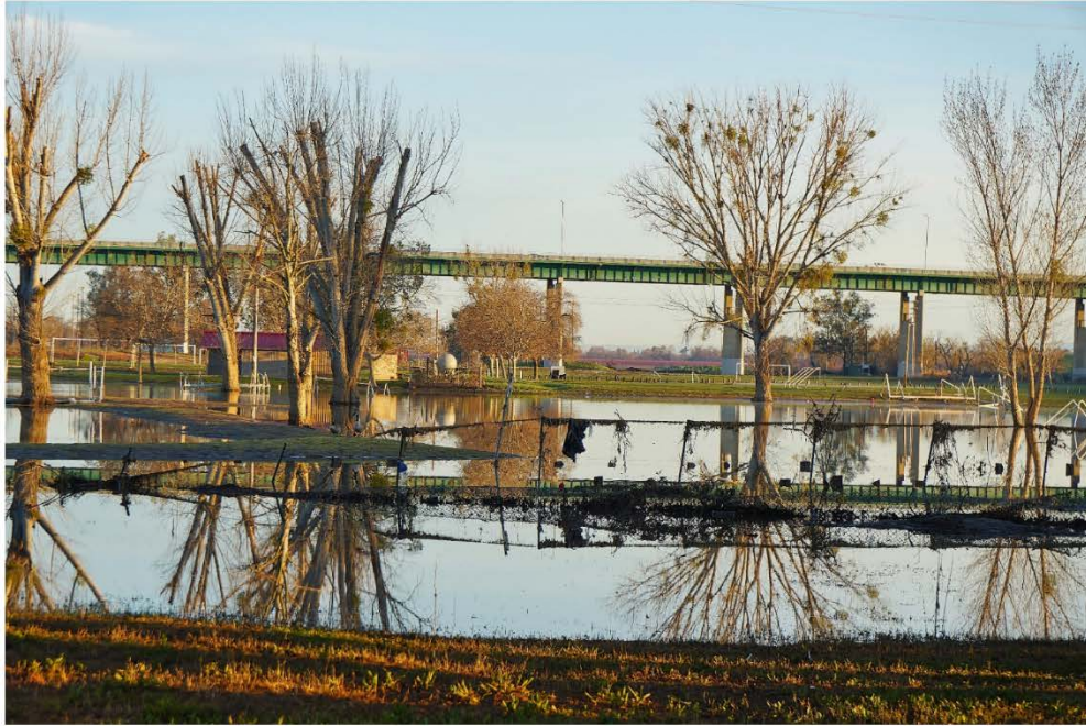
Photo 02: South side of levee after Oroville Dam release in phase 2A
