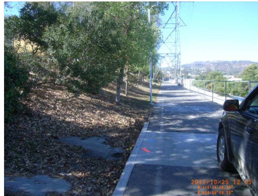
Photo 4: Looking upstream near downstream end of LAR 3. Not a levee condition. Ascending slope to high ground on landside. Vegetation would be within the VFZ if this portion is to remain listed as levee or is required for levee support upstream or downstream.
