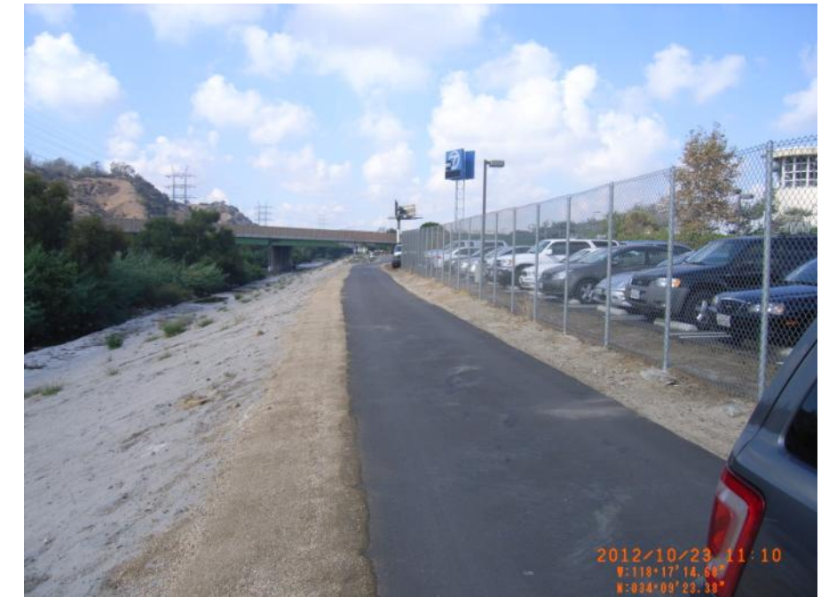
Photo 17: Looking upstream on LAR 7. Landside backfilled and not a levee condition.
