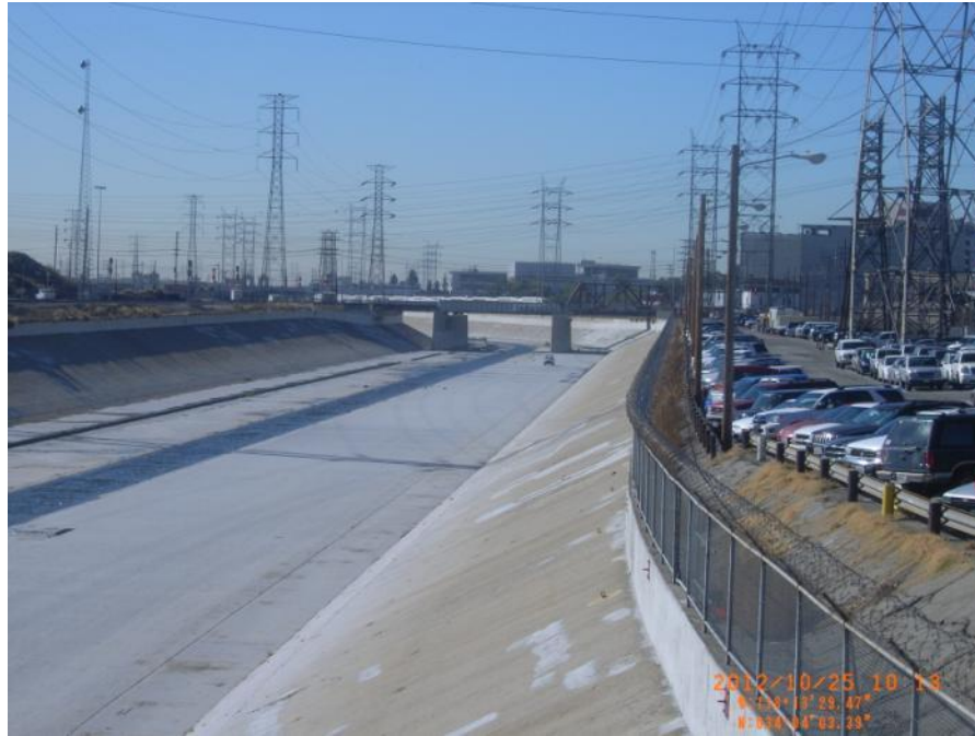
Photo 1: View looking downstream at N. Main Street. LAR 2 on right side. Not a levee condition. From top of wall and ascending slope approximately 5-feet in height with relatively level ground on landside.
