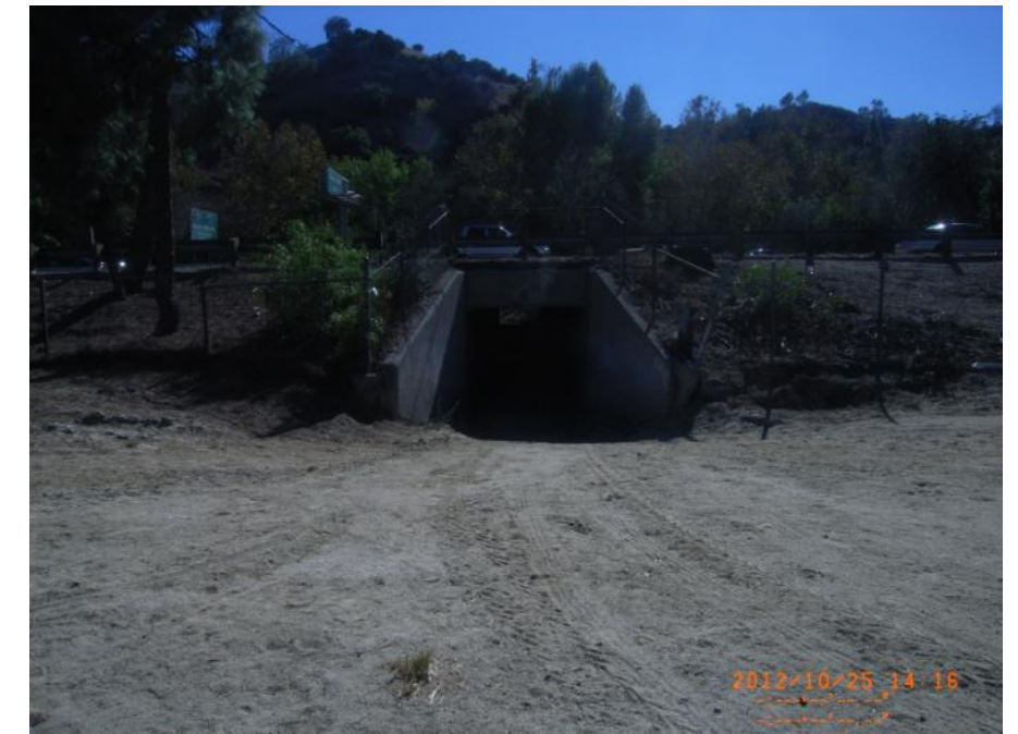
Photo 12: Equestrian undercrossing on landside of LAR 3. Photo taken at landside crest.
