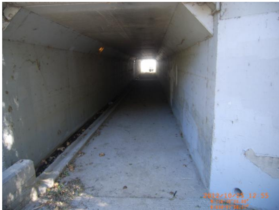
Photo 8: Landside of tunnel culvert at end of tunnel in background. Tunnel height allows horse and rider to pass through without rider bending over. Note small wall in foreground as it is the same wall depicted in Photo 9.
