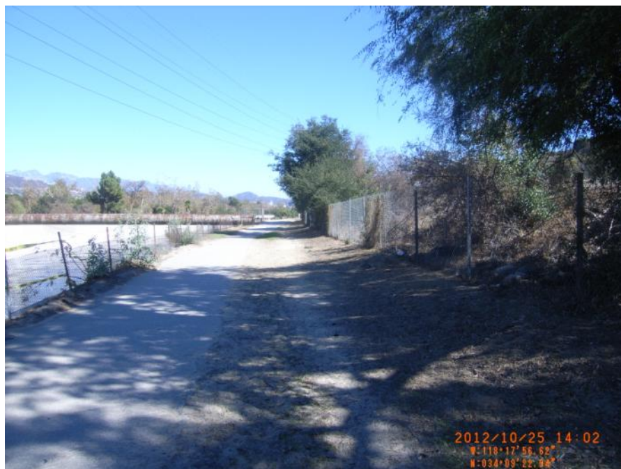
Photo 14: Upstream end of LAR 3 looking downstream. Vegetation on landside.
