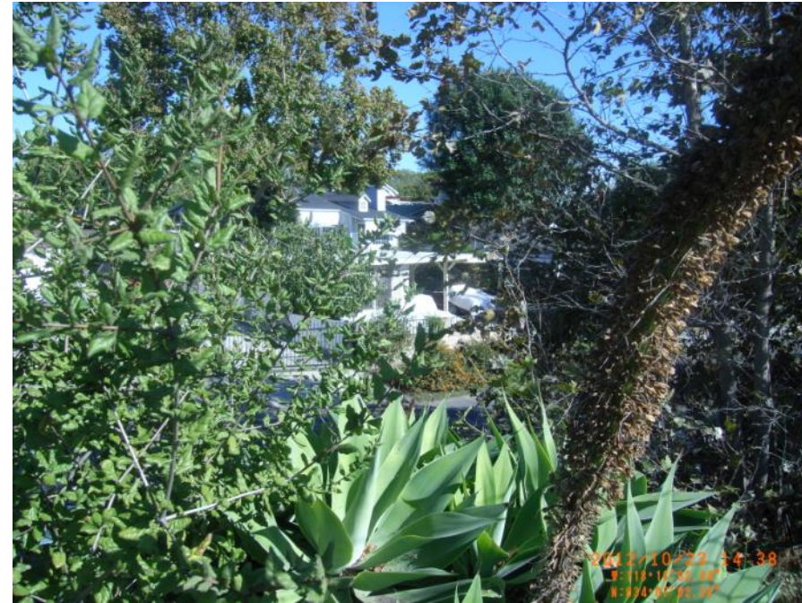
Photo 21: Vegetation on landside and levee condition on LAR 6.
