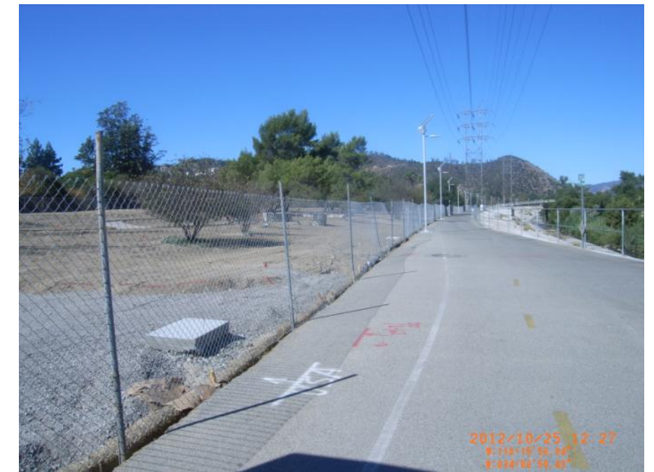
Photo 6: Looking upstream along LAR 3 just upstream of Hyperion Ave. Not a levee condition. Grades for park are above crest.
