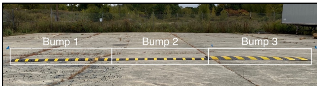
Figure 2. Speed bumps installed on the concrete pad referenced in Fig. 1.
