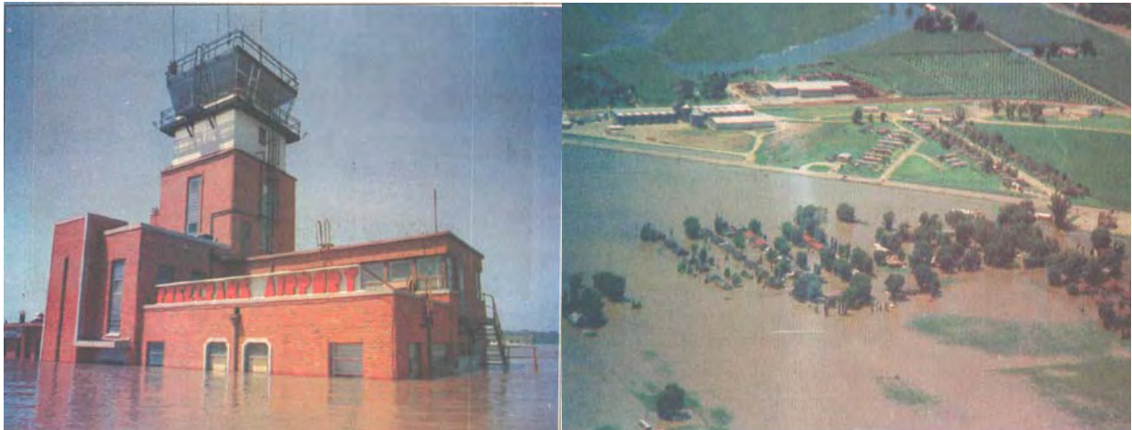
Clockwise from top left: Looking west where U.S. Highway 36 crosses the Missouri River and disappears into flooded Elwood, Kansas; floodwaters surround the St. Joseph water treatment plant; floodwaters in Wathena, Kansas; Rosecrans Memorial Airport terminal building.
