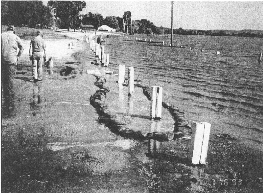
Figure 8. Ringed Sand-boils during Flood of 1993.
