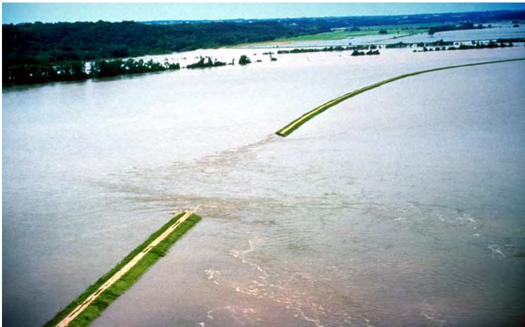
Figure 3 – Breach of Unit R471-460 during and after the Flood of 1993
