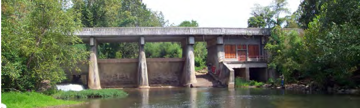
Figure 12. Lake Craig Dam Existing Conditions
