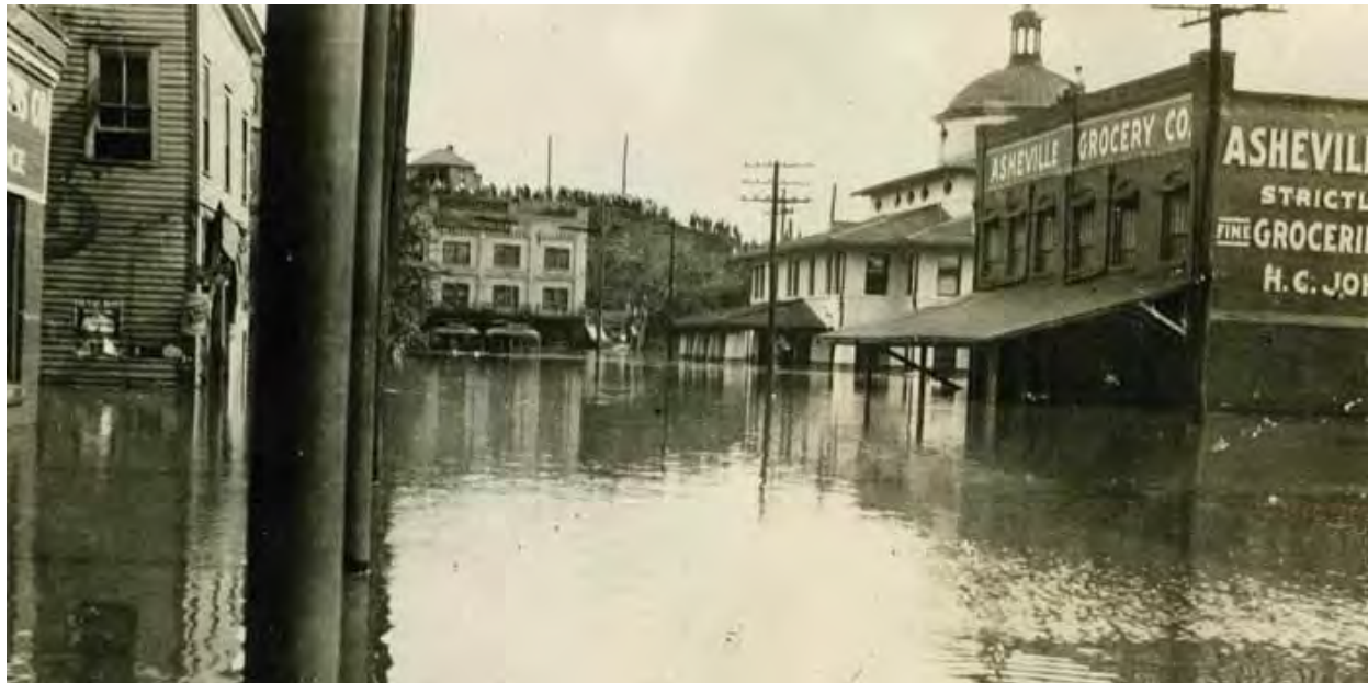
Figure 5. City of Asheville, July 1916 Flood
