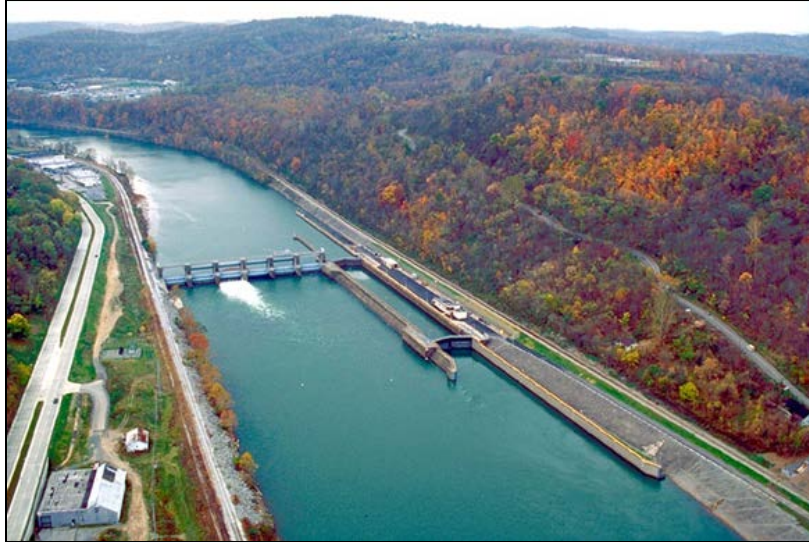
Figure 4. Morgantown Lock and Dam.
