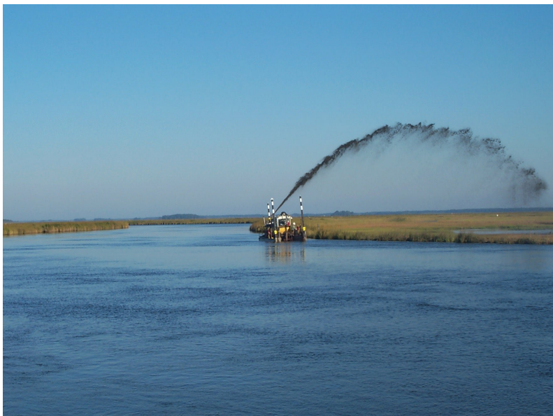
Figure 2. Spray disposal of dredged material (photograph courtesy of Bob Blama, CENAB, USACE)
