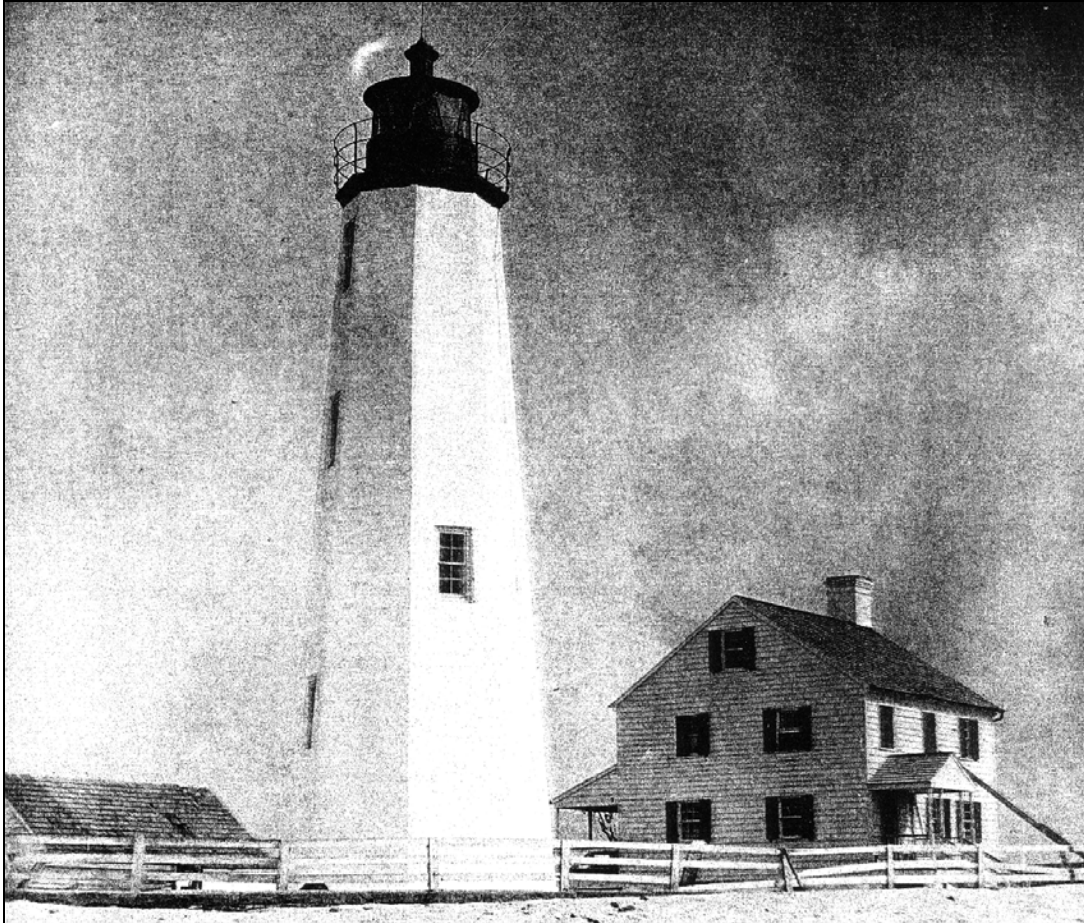
Figure 66. New Point Comfort Lighthouse, Mobjack Bay, Mathews County, Virginia (Photograph courtesy of the Maryland Historical Trust, Crownsville, Maryland).
