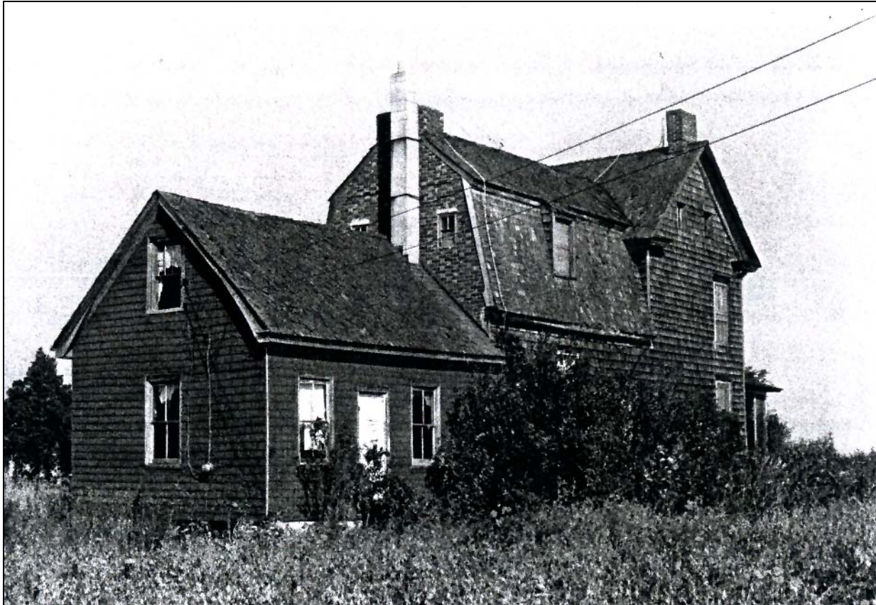
Figure 27. Opposing view of the Lewis Landing House (DO201) located in Dorchester County has been nominated to the NRHP (Photo courtesy of the Maryland Historical Trust).
