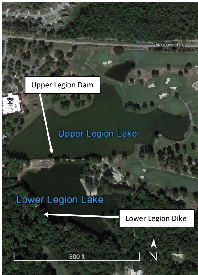
Figure 1.6 – Upper and Lower Legion Lakes Post Emergency Repair.
