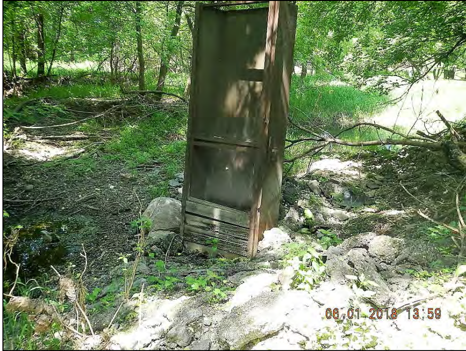
Figure 9. General view of abandoned stoplog structure
