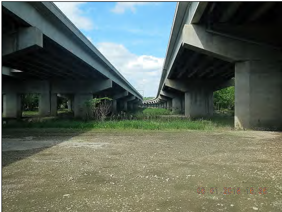
Figure 50. General view looking north across parking lot beneath US Highway 169
