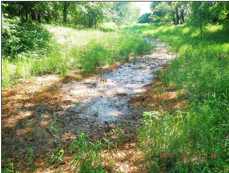
Figure 30. Looking upstream of iron pipe inlet
