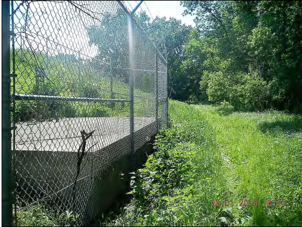
Figure 35. Southern property boundary of Blue Lake Treatment Plant looking east
