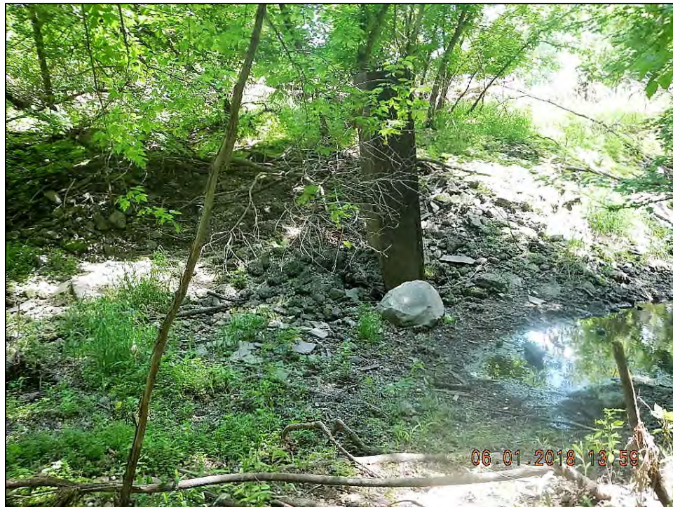
Figure 10. View of abandoned stoplog structure looking towards Cargill
