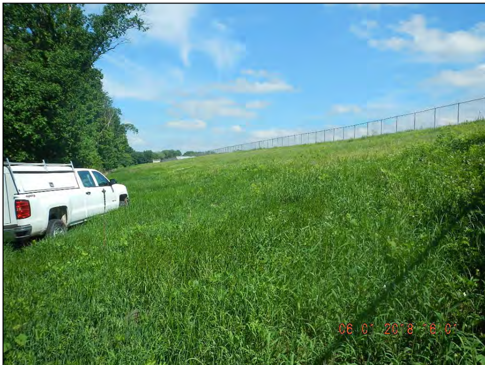
Figure 36. Southern property boundary of Blue Lake Treatment Plant looking west
