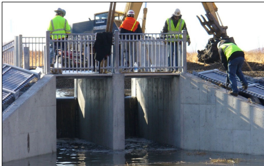
Figure 3: Long Meadow Lake Water Control Structure During Handrail Construction
