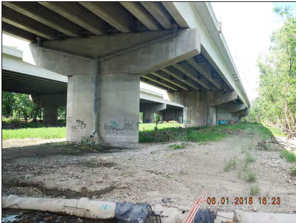
Figure 48. General view looking north along US Highway 169
