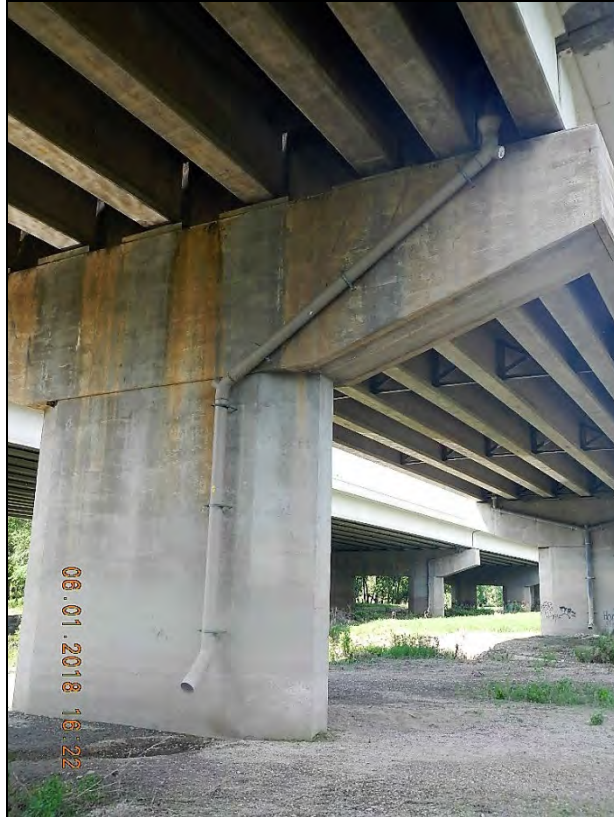
Figure 45. US Highway 169 roadway drainage discharge pipes
