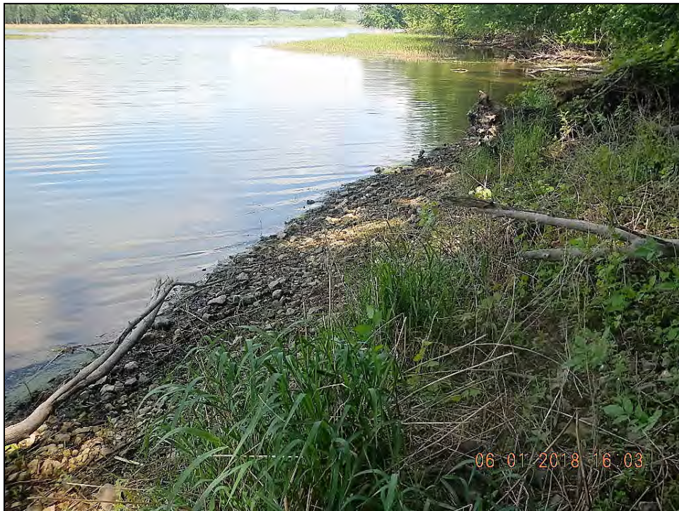
Figure 38. Man placed riprap along southern shore of Blue Lake
