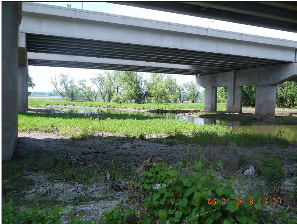
Figure 40. Fischer Lake outlet channel under US Highway 169
