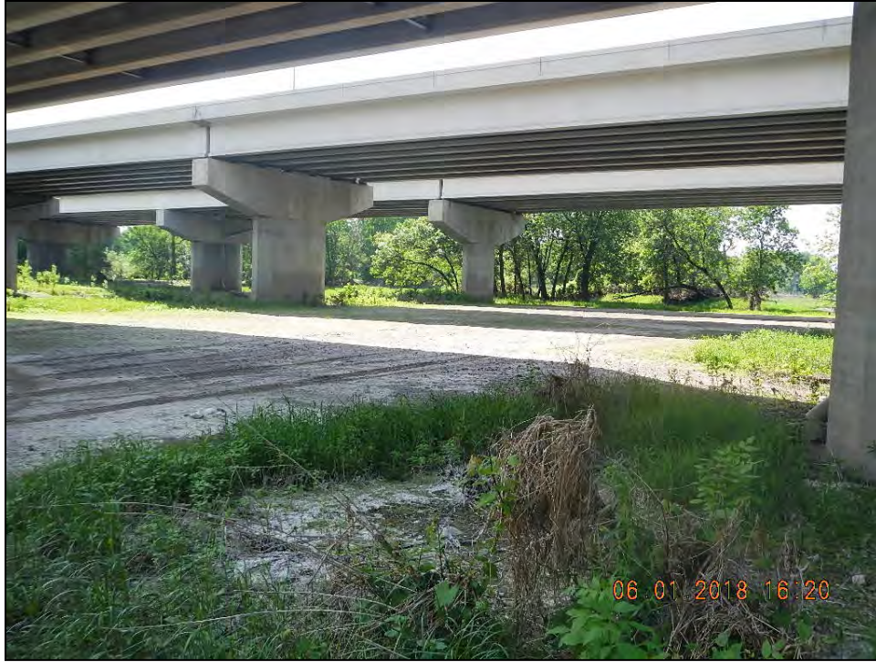
Figure 39. Gravel parking lot under US Highway 169
