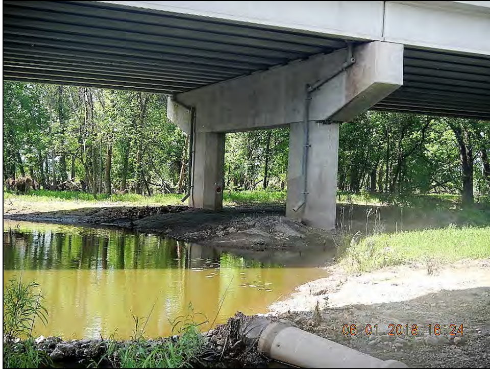
Figure 49. Southbound bridge pier of US Highway 169
