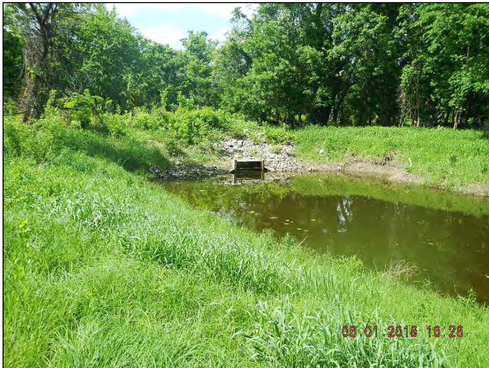
Figure 52. Rice Lake EMP West outlet stop log structure
