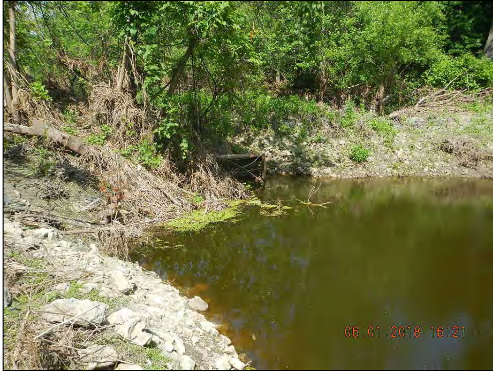
Figure 43. Rice Lake outlet structure
