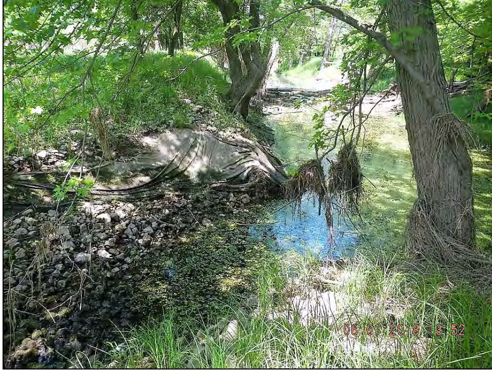
Figure 3. Geotextile and riprap within stoplog bypass channel
