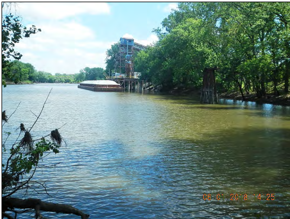
Figure 18. Cargill barge loading facility and harbor
