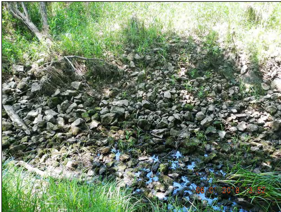
Figure 4. Riprap within stoplog bypass channel
