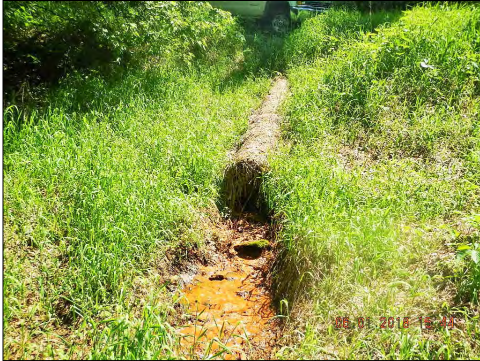
Figure 27. Discharge end of 12-inch iron pipe under Blue Lake refuge trail
