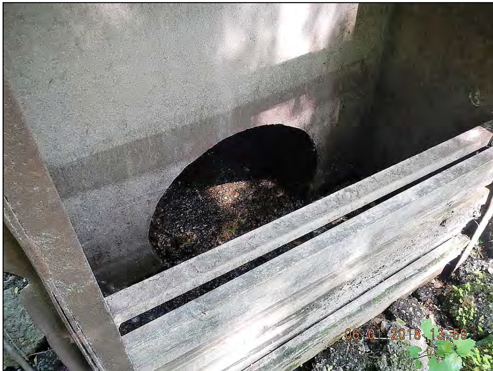
Figure 8. View inside of stoplog structure
