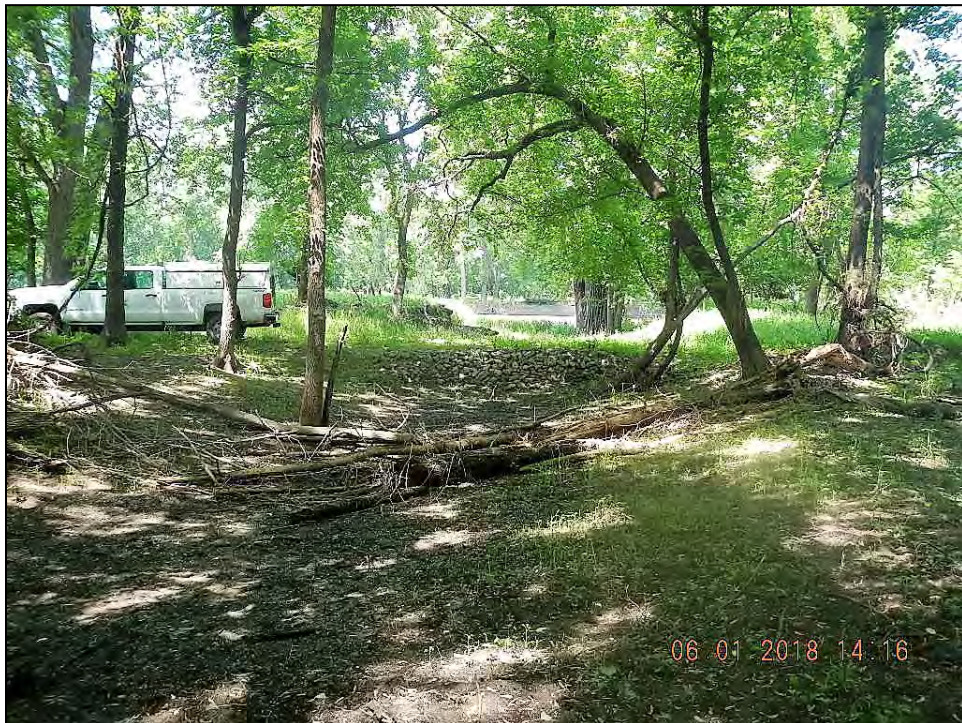
Figure 16. Downstream view of rock spillway structure
