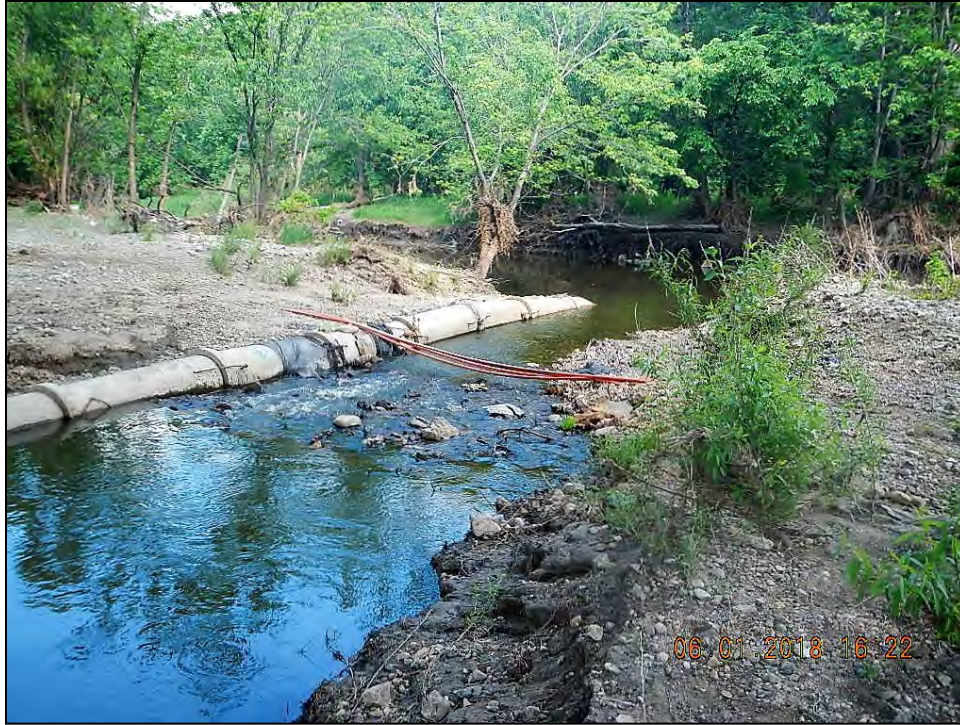
Figure 47. Scour channel and miscellaneous utilities traversing site
