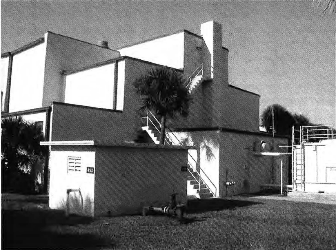
Figure 33. Electrical Substation, Building 453.
