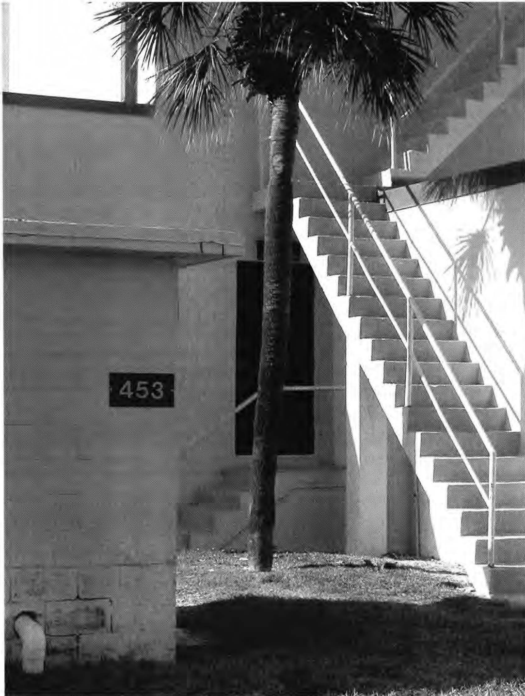
Figure 6. L-shaped Exterior Stairs to Fan Room.
