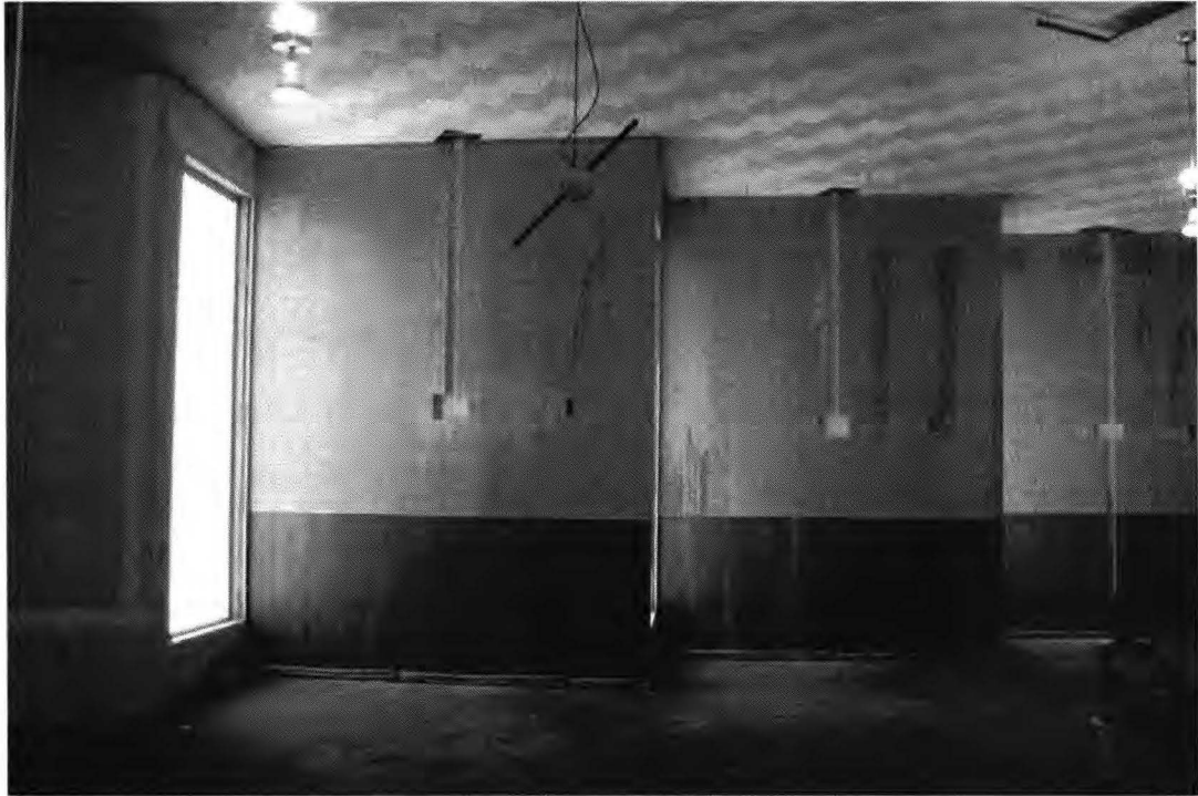
Figure 14. Interior View of Nave Stepped Sidewalls. (Martin Stupich, 2004)
