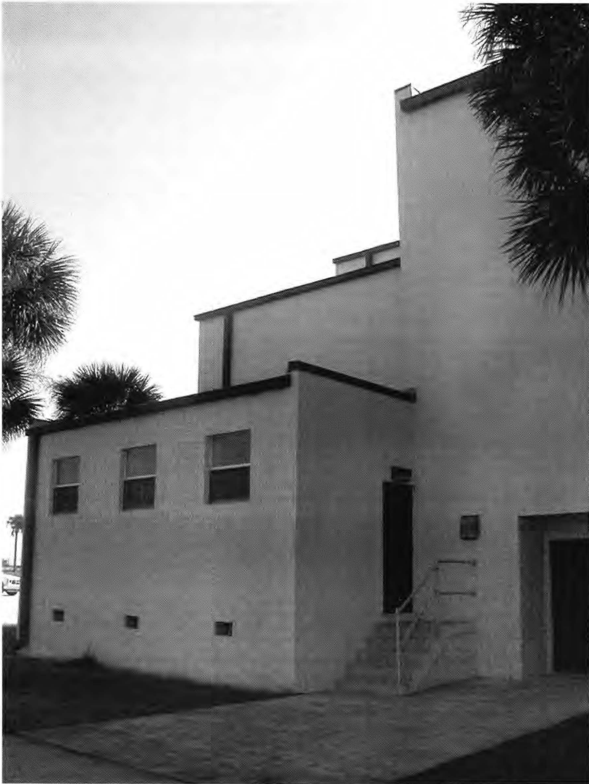
Figure 9. Typical Dressing Room Exterior Access Door.
