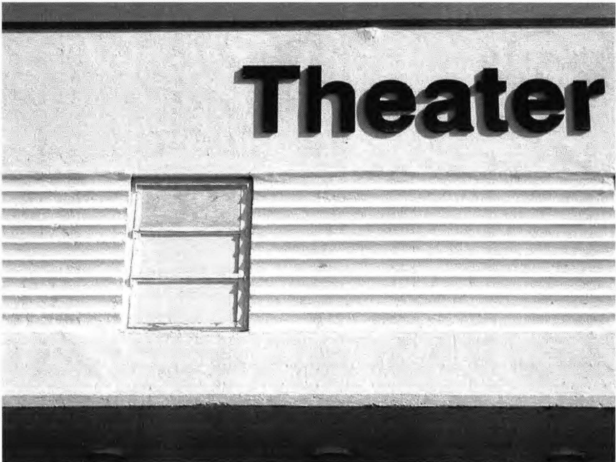
Figure 3. Art Deco Fluted Stucco Panels.
