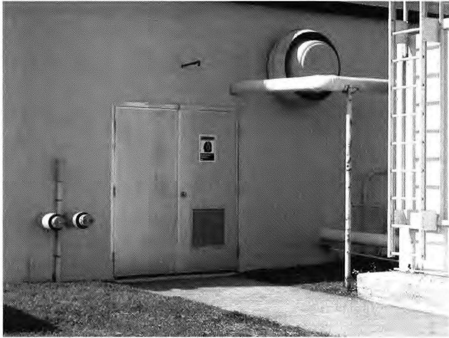
Figure 10. Equipment Room Exterior Access Door.
