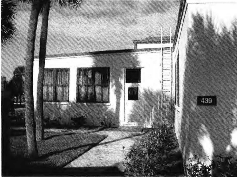
Figure 12. Typical Replacement Fixed Transom Over Door.
