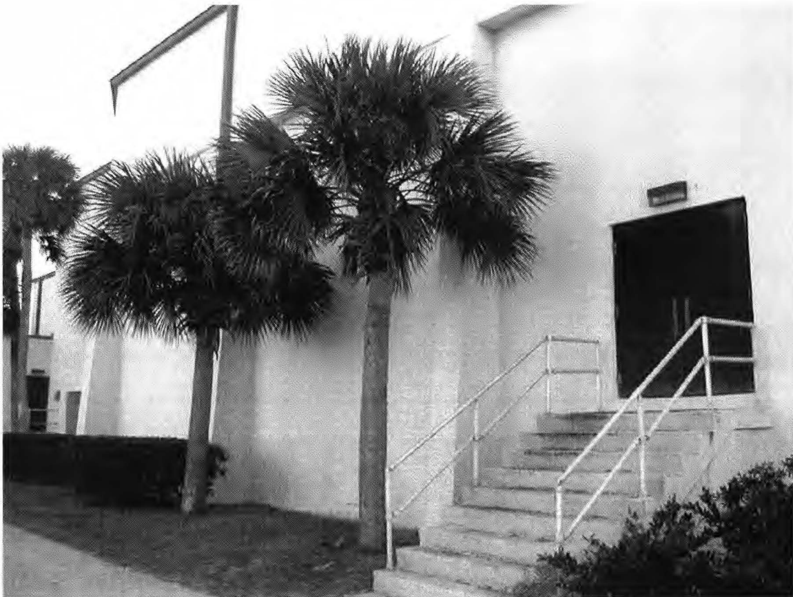
Figure 5. Exterior Egress Stairs at Auditorium.
