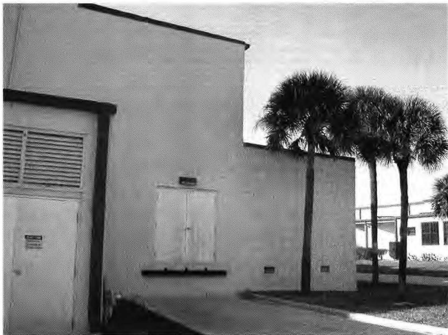
Figure 11. Stage Equipment Doors/Loading Dock.
