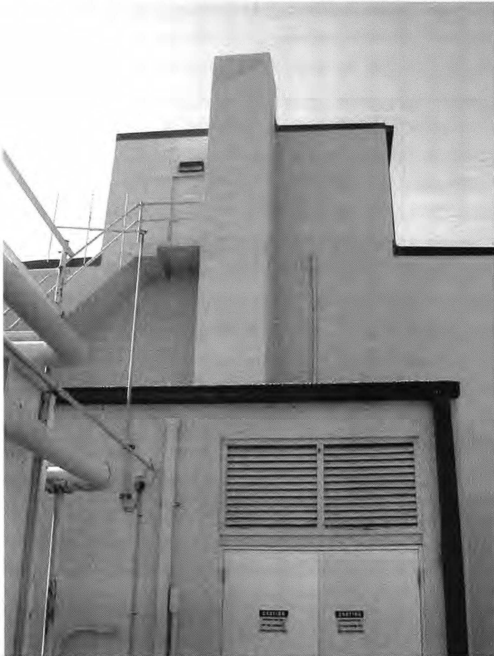
Figure 14. Original Boiler Room Louvered Vents.
