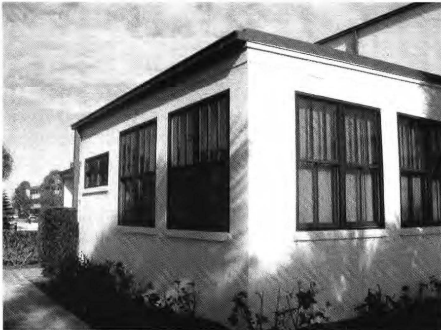
Figure 13. Typical Replacement Anodized Aluminum Windows.
