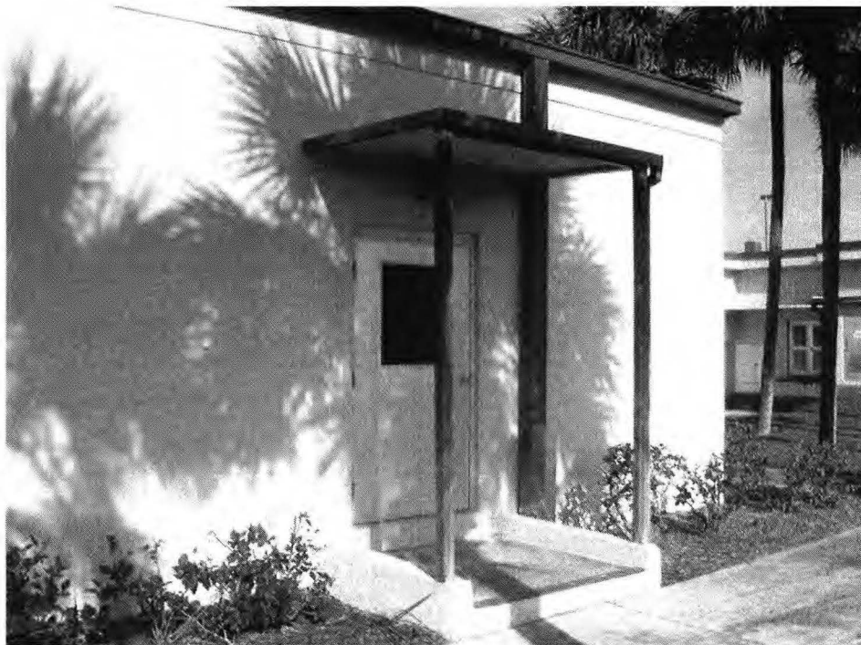
Figure 9. Modified East (Rear) Entry Porch.
