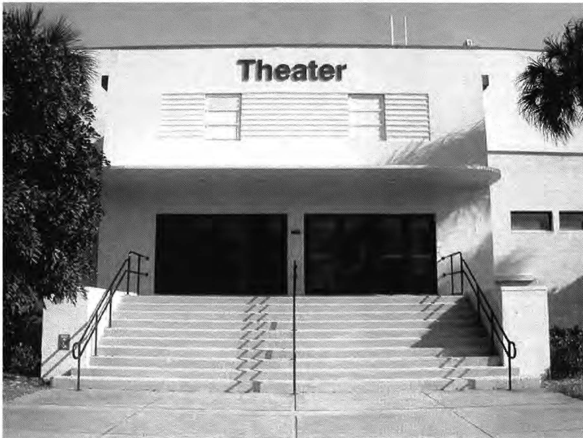
Figure 8. Front Entry Doors.
