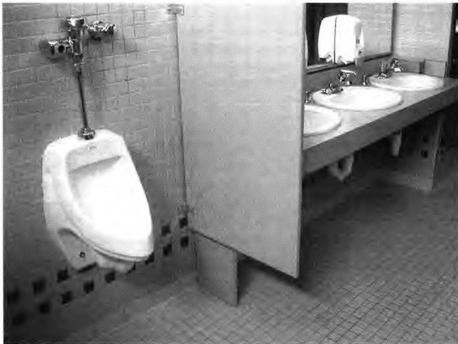
Figure 28. Lavatories, Wing Wall, and Urinals in Men's Restroom.
