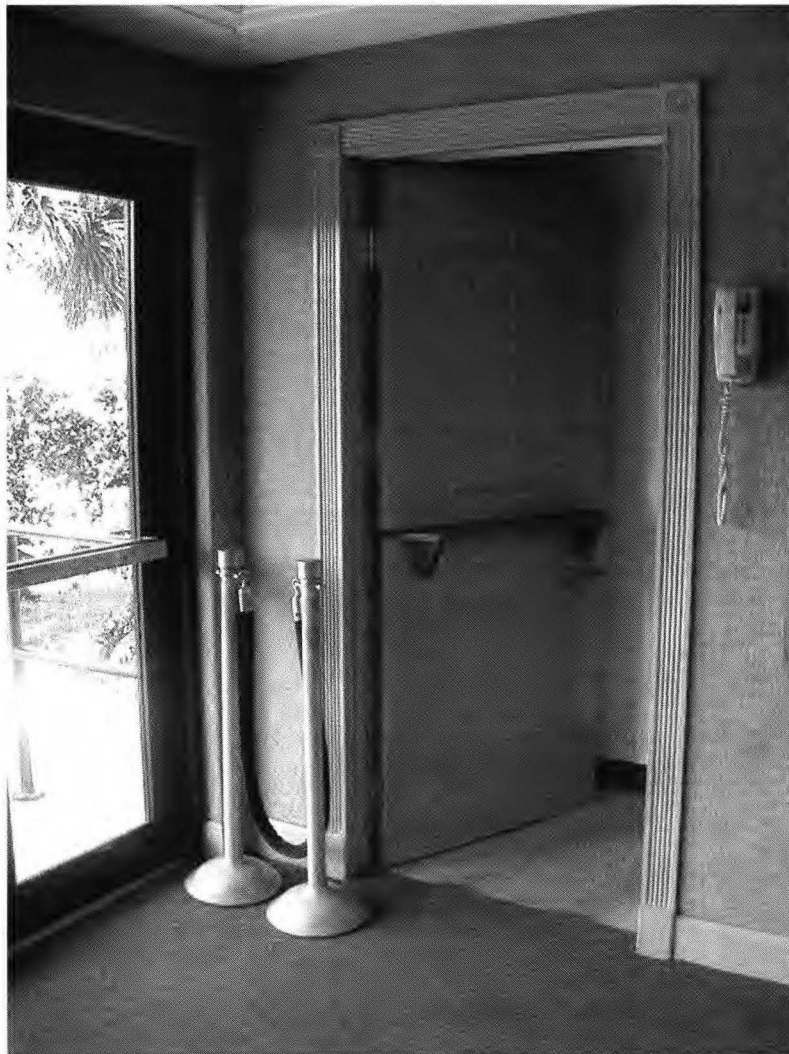
Figure 20. Lobby Ticket Booth Dutch Door.
