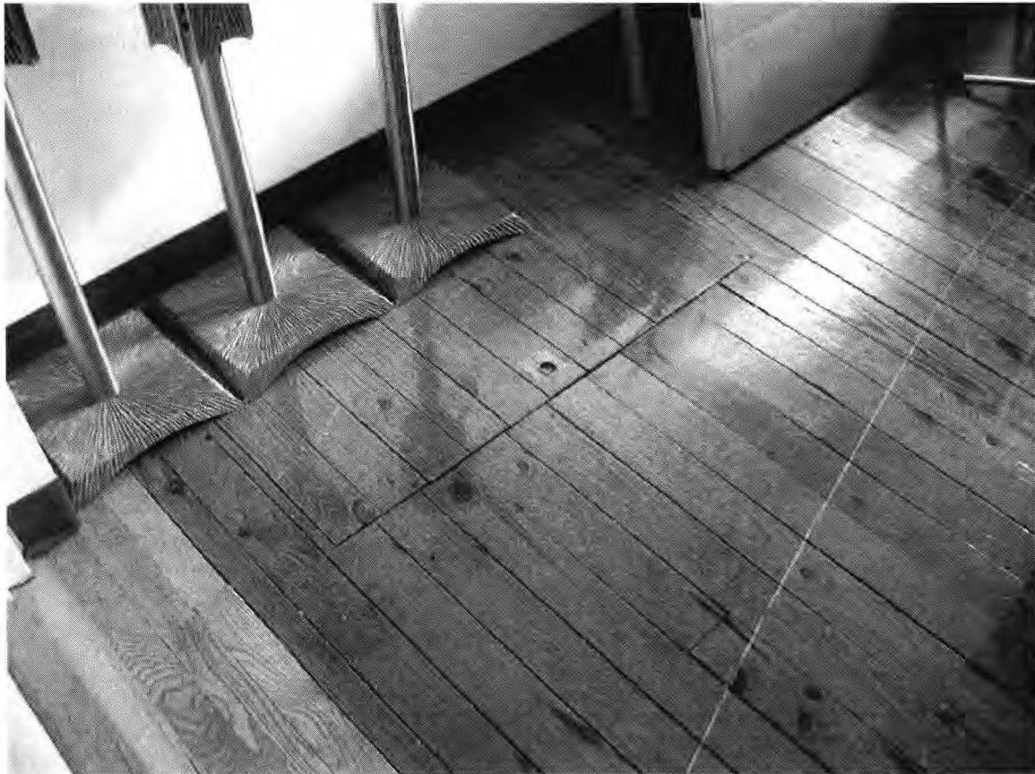
Figure 18. Original Crawlspace Access Hatch in Floor.
