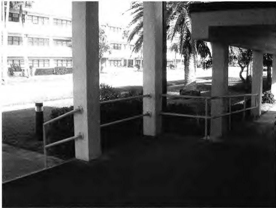
Figure 8. Covered Walk Canopy to Building 440 Adjoins Building 439 Entry Portico.
