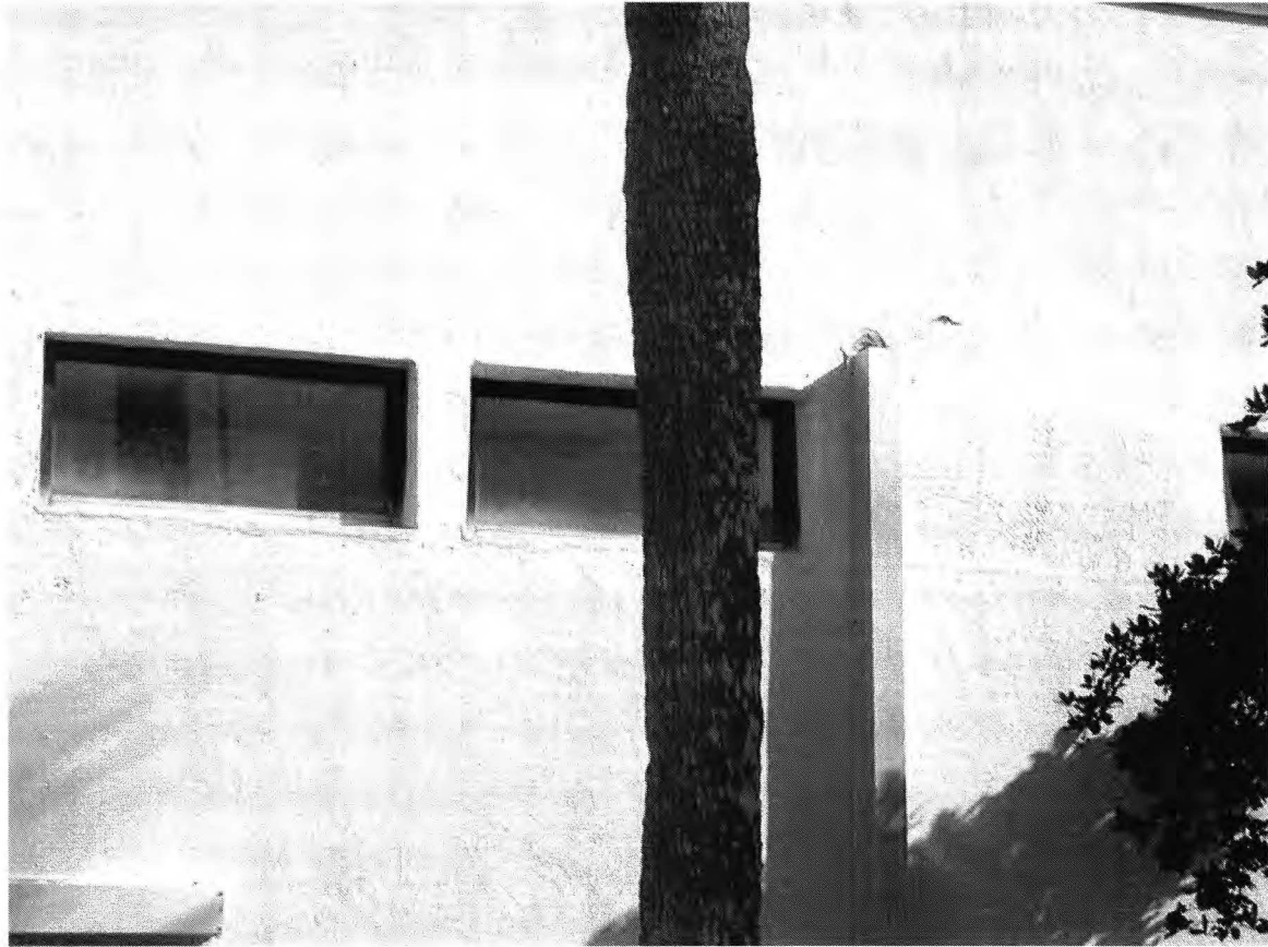
Figure 13. Blocked Window Opening Covered in Stucco (right).
