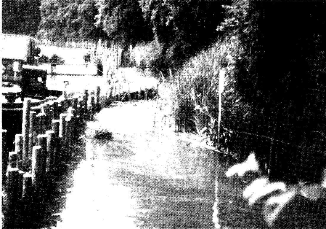
Figure 4. Poles that are initially placed with a jetpump
