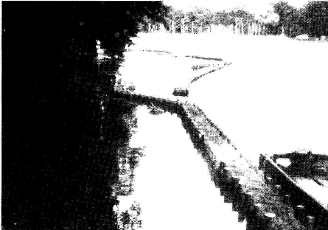
Figure 5. Completed branchbox breakwater
