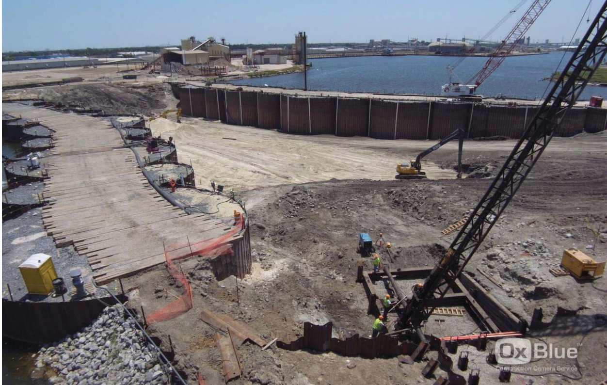
Figure 2. Seabrook Cofferdam unwatered May 5, 2011.
