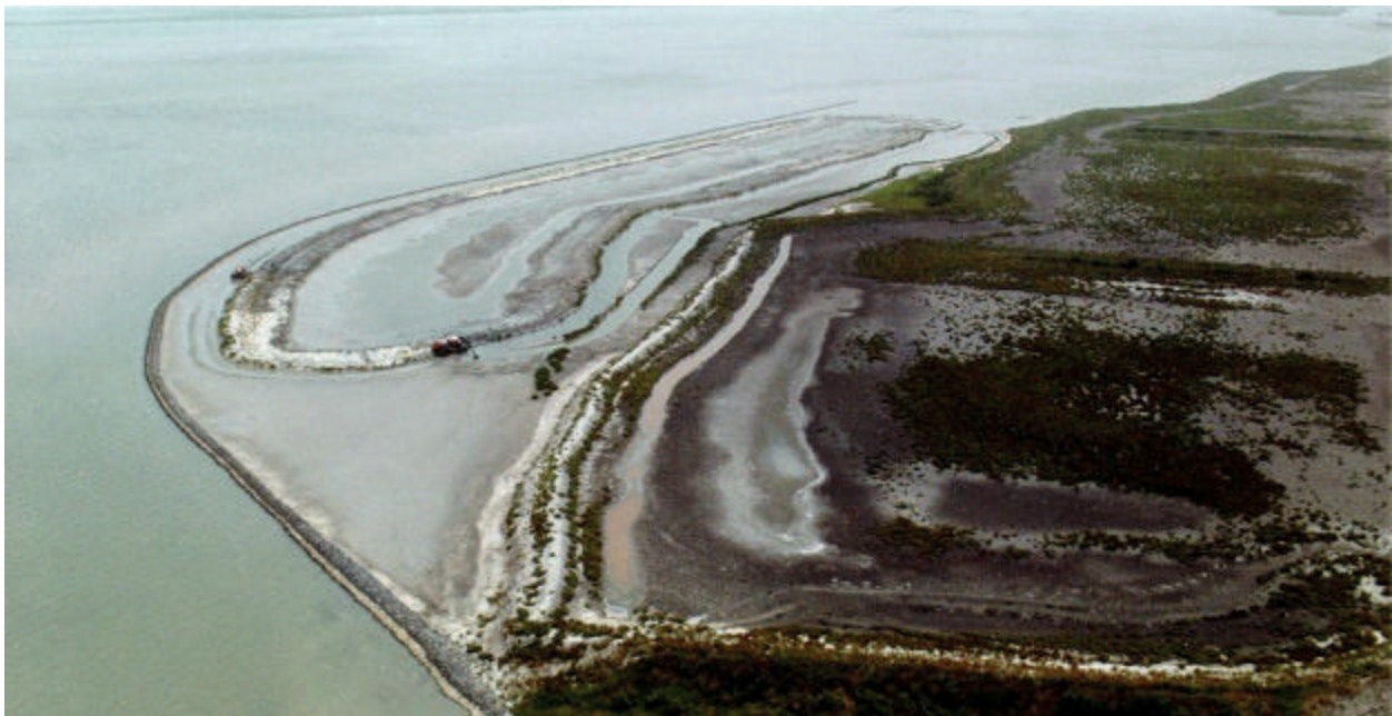
Figure 1. Riprap breakwater used to reduce wave energy reaching a created salt marsh
