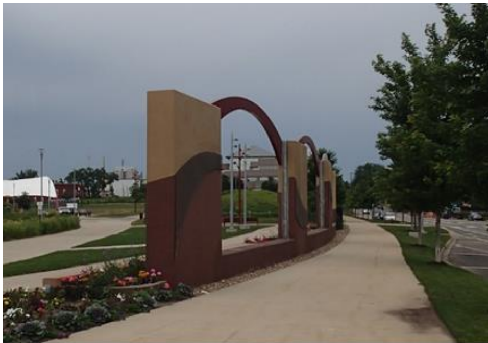
Figure 6. Combination wall near the Cedar Rapids amphitheater.
