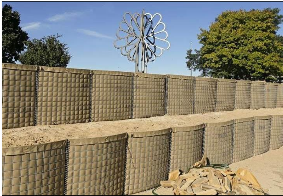
Figure 15. Hesco barrier system deployed at Cedar Rapids, IA (photo: Stephan Mally/ The Gazette ).
