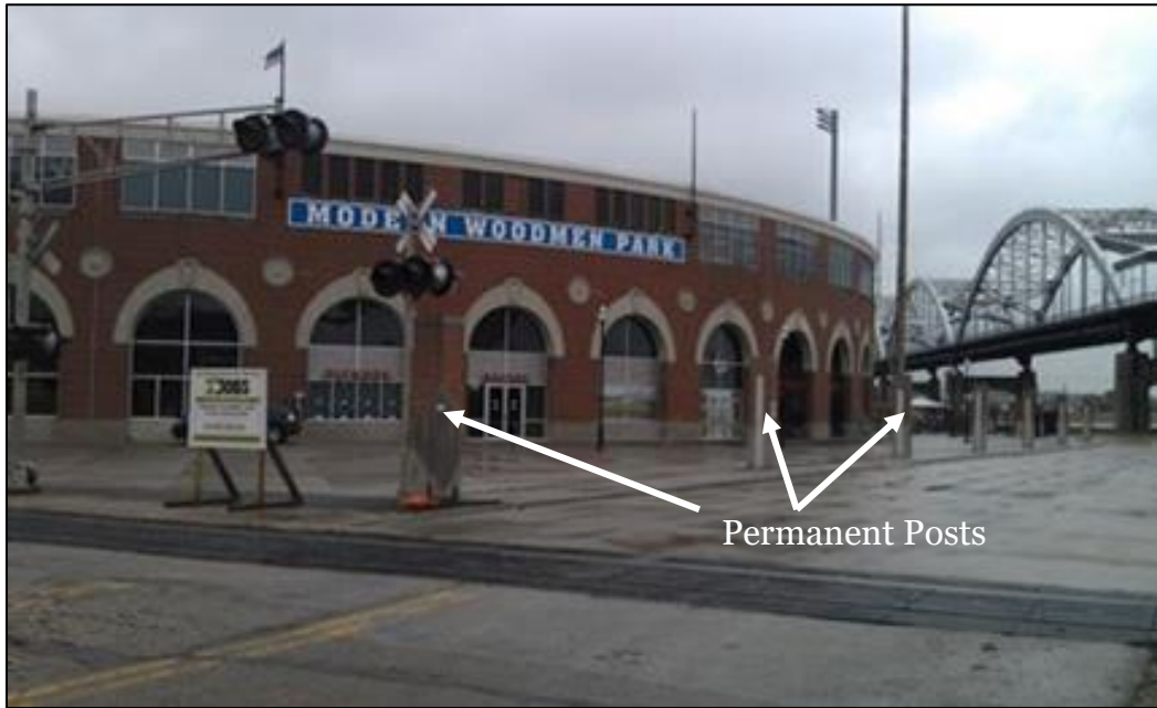
Figure 7. Combination wall in Davenport, IA, before deployment.
