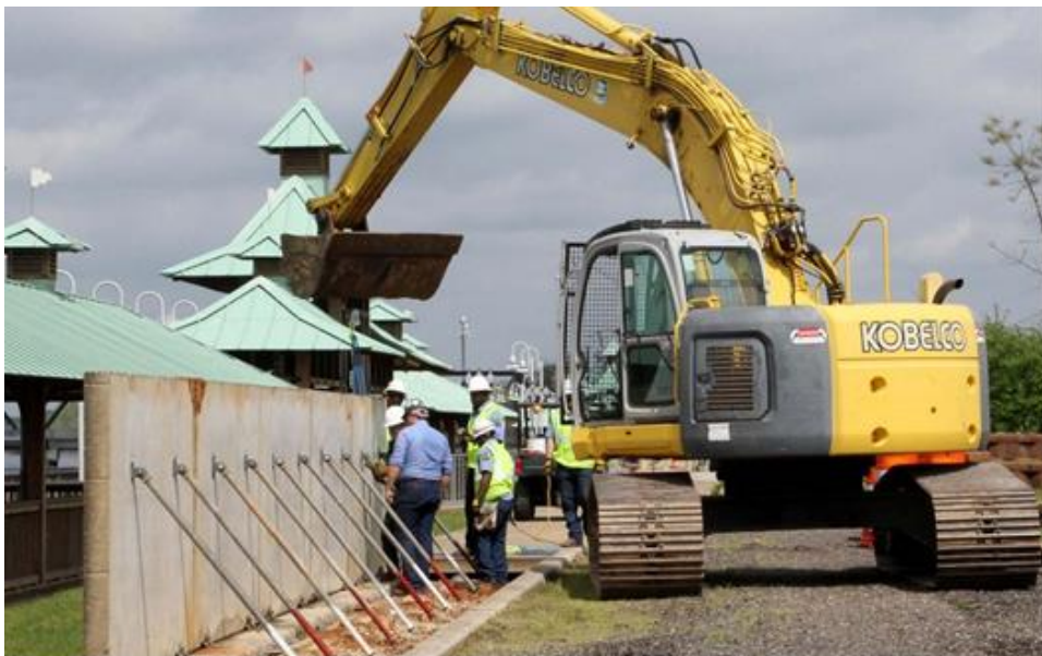
Figure 5. Monroe Solution floodwall being put in place.
