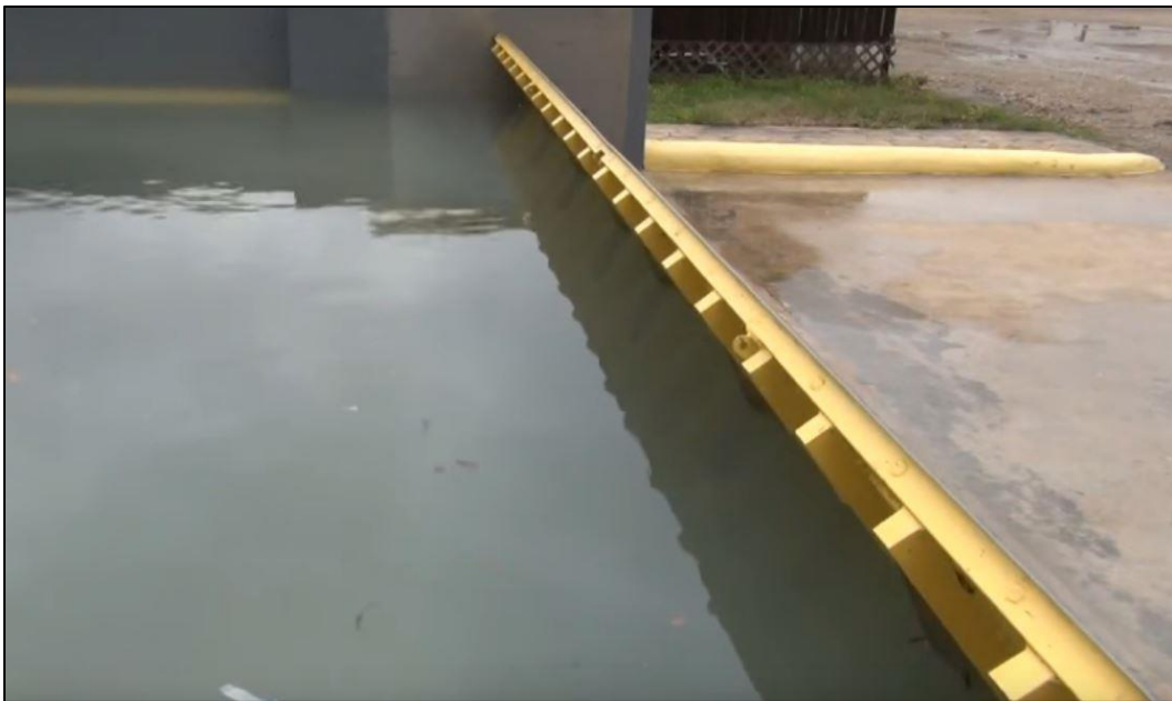
Figure 13. Pop-up gate (photo: FloodBreak®).
