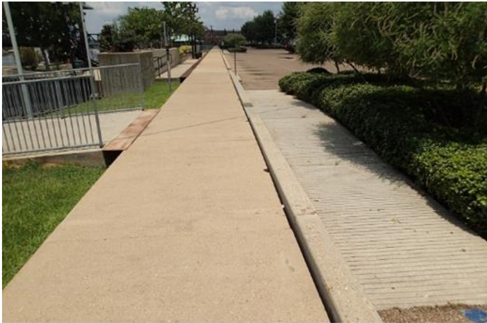
Figure 4. Monroe Solution floodwall in sidewalk position.
