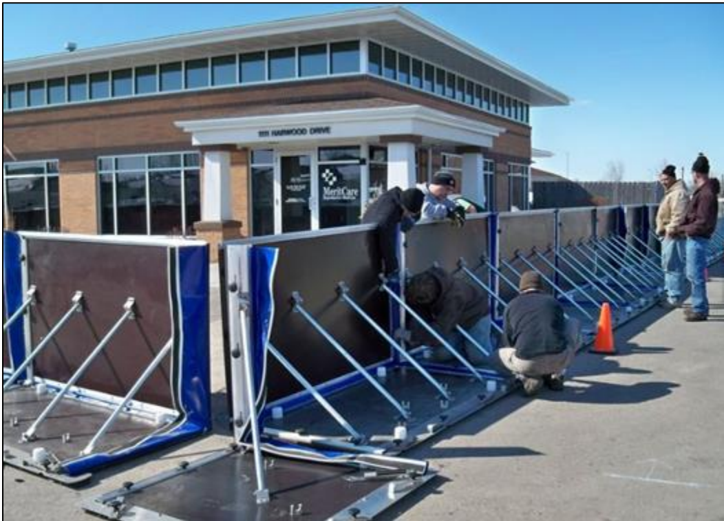
Figure 14. Aquafence installation.
