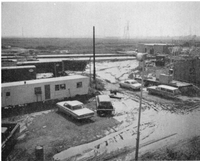
b. Flooded sewage treatment plant
