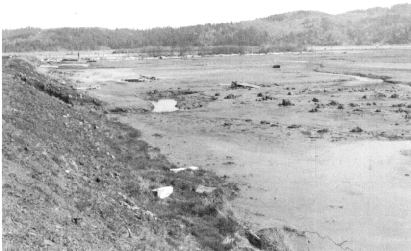
b. Debris on tidal flats downstream of failed sluice structure
