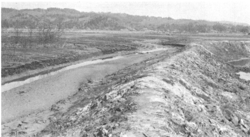
Fig. 37. Borrow ditch (at left of dike) for dragline-constructed dike (Portland District)
