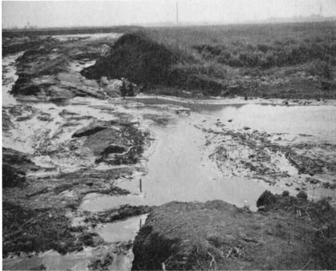
a. A 150-ft-wide break in the 20-ft-high dike section
