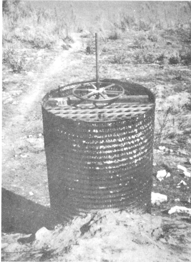
Fig. 14. Flood control valve on exterior side of sluice discharge pipe
