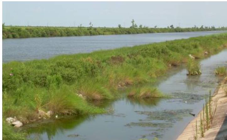
Photo 1. East Bank of Parish Line Canal (looking northwest)
