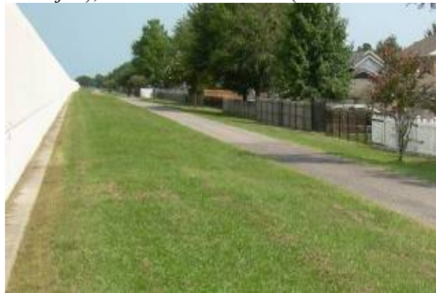
Photo 2. Example habitat on protected side of existing floodwall
