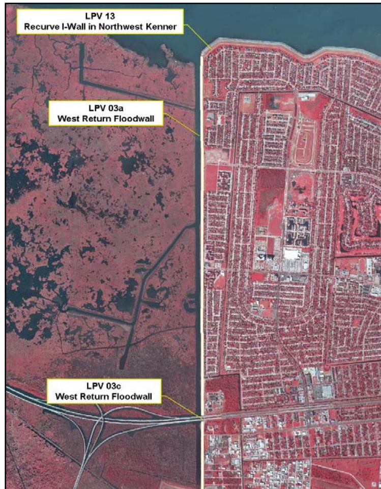
Figure 2. IER # 2 - West Return Floodwall Jefferson and Recurve I-Wall Kenner
