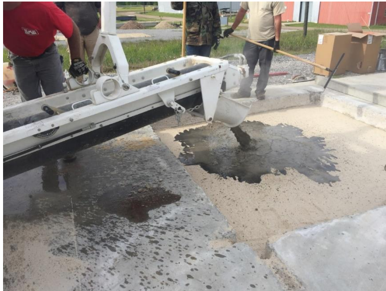
Figure 28. Excessive water initially delivered from volumetric mixer.
