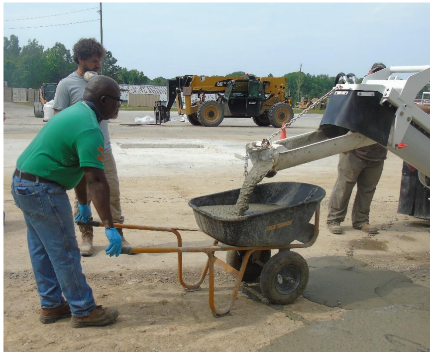
Figure 21. Sampling freshly mixed concrete.
