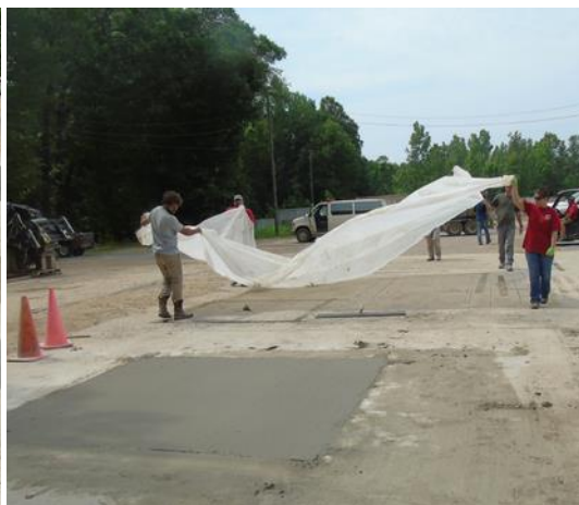
(f) Covering test section with plastic
