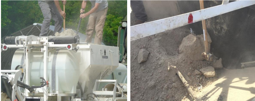
Figure 27. Large portions of compacted MPC material being broken down.
