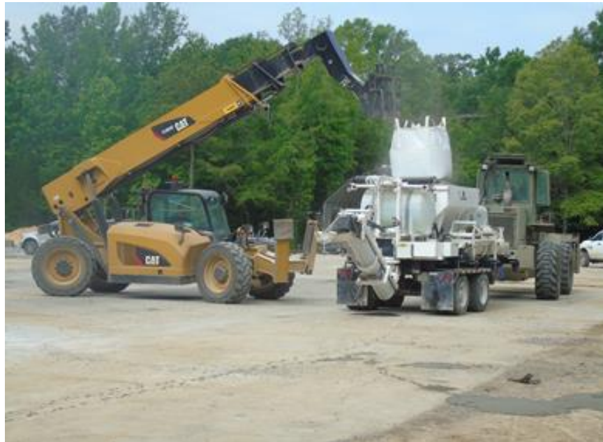
Figure 20. Loading the volumetric mixer for concrete placement of MPC materials.
