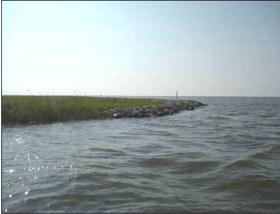
Figure 2-18. Example of Onshore Placement of Rock for Shoreline Protection
