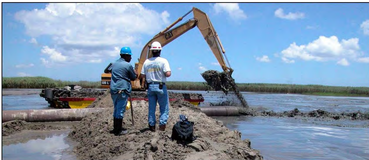
Figure 2-16. Dredge Material Placement for Marsh Restoration
