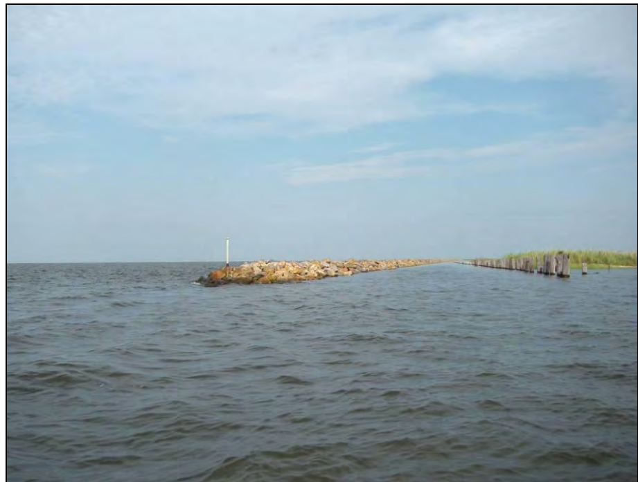
Figure 2-19. Example of Offshore Placement of Rock for Shoreline Protection
