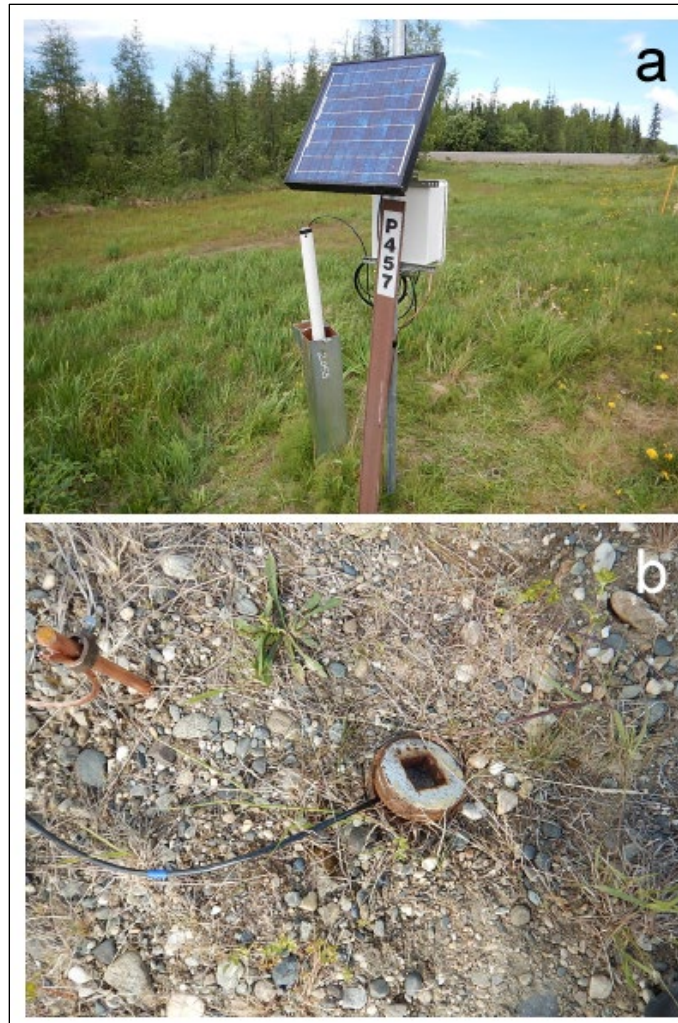
Figure 6. An example of frost jacked PVC casing (a), the piezometers located along the top of the embankment are flush to the ground surface, where rocks and dirt can easily be pushed into the piezometer (b).
