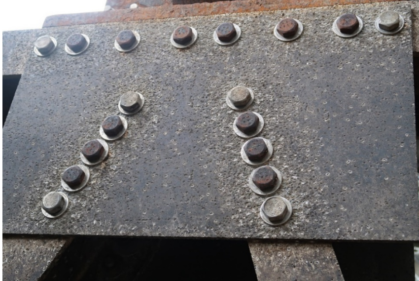
Figure 12. Montgomery aluminum bulkhead after power washing.
