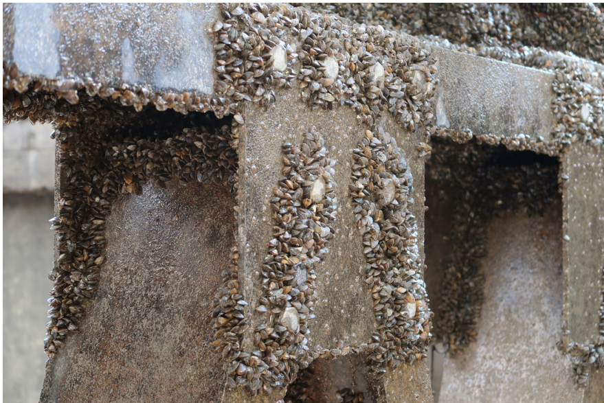
Figure 10. Zebra mussels on Montgomery aluminum bulkhead (image 1).
