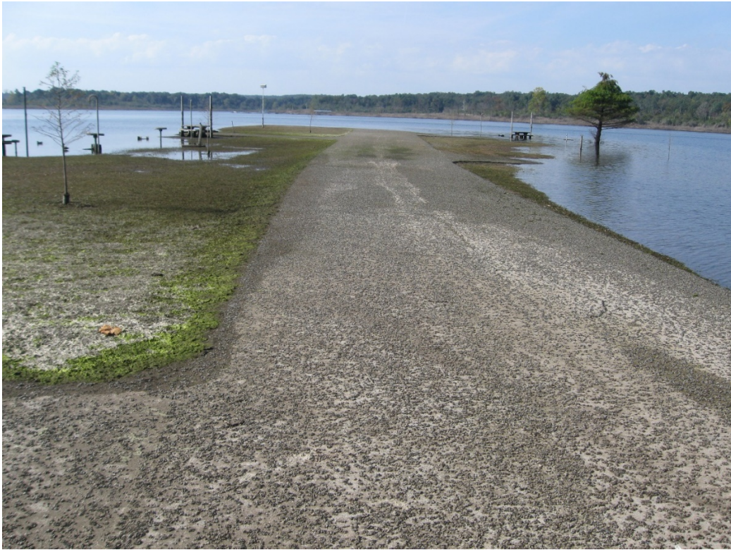
Figure B-5. Lead Hill Park boat ramp 2015, Little Rock District.
