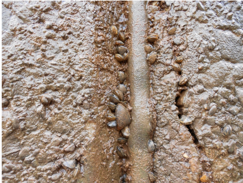
Figure B-1. ZM on concrete in lock chamber of #3 Lock & Dam on Red River, April 2017, Vicksburg District.
