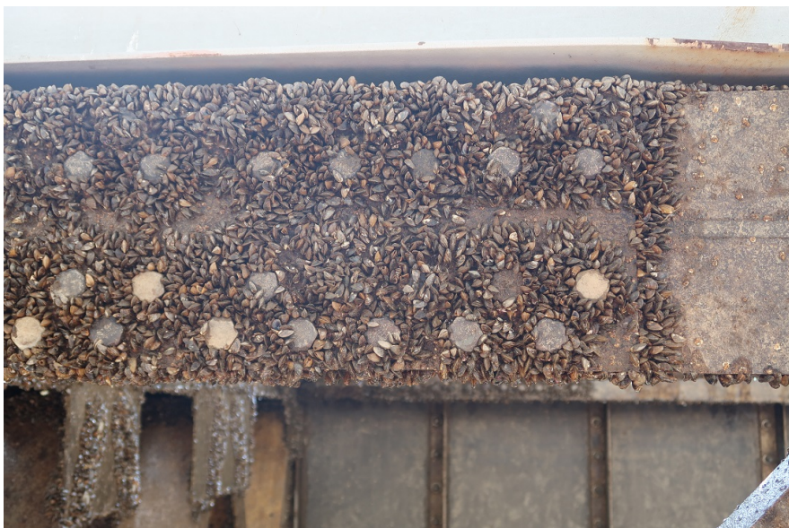
Figure 11. Zebra mussels on Montgomery aluminum bulkhead (image 2).
