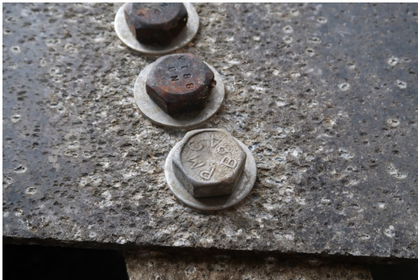
Figure 13. Montgomery aluminum bulkhead after power washing (closeup).
