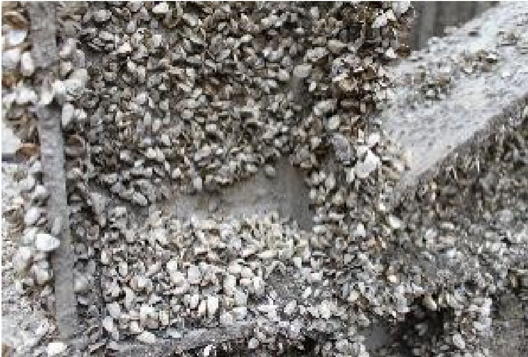
Figure 1. Zebra Mussels on sector gates at T.J. O'Brian Lock & Dam, Rock Island District 2015.
