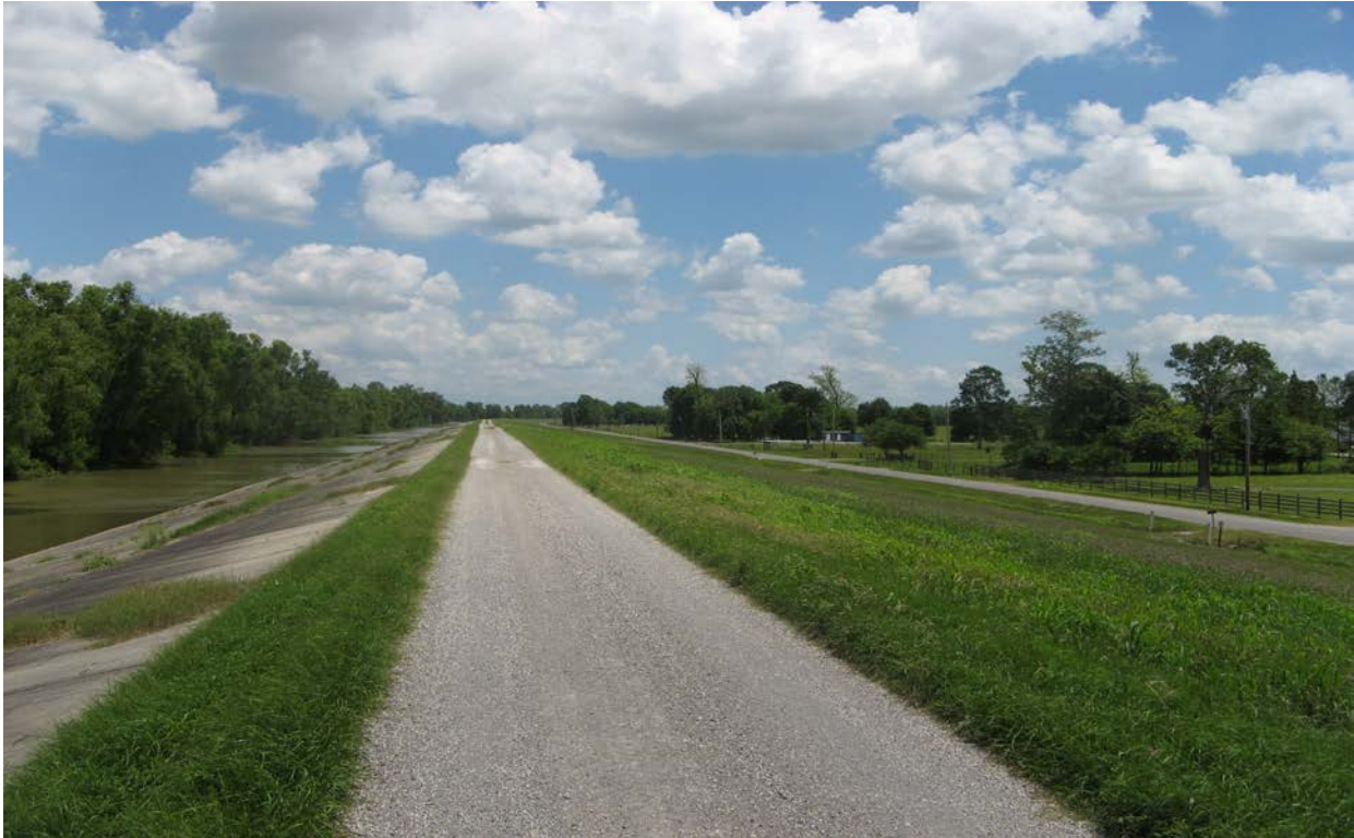
Figure 5. Mississippi River levee – St. Gabriel levee site existing conditions.
