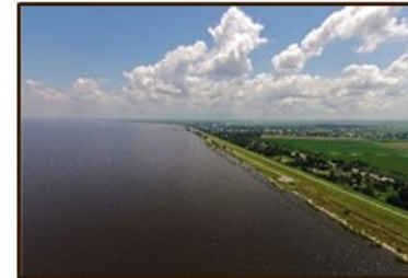
Lack of vegetation/habitat along Lake Okeechobee's southeastern shoreline
