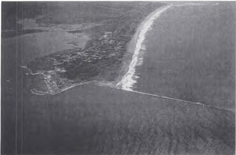
Photo 8. Looking south, May 1994 (Photo courtesy of City of Westport)
