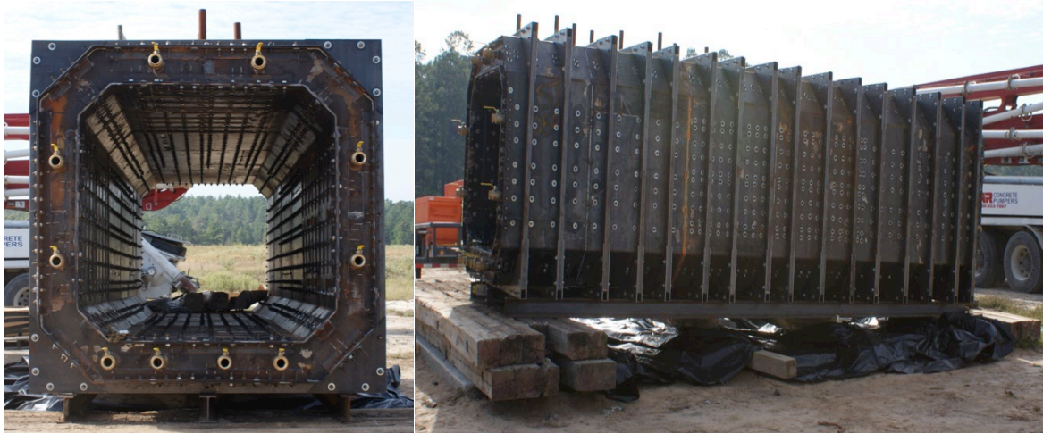
Figure 2. The 7 ksi column cross-section (left) and inclined steel formwork (right).
