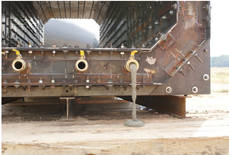
Figure 7. Grout flowing through the first ball valve located on the inclined side.
