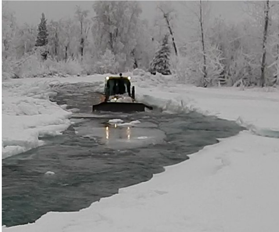
Figure 9. Bulldozer removing ice from the channel bed (January 2017).
