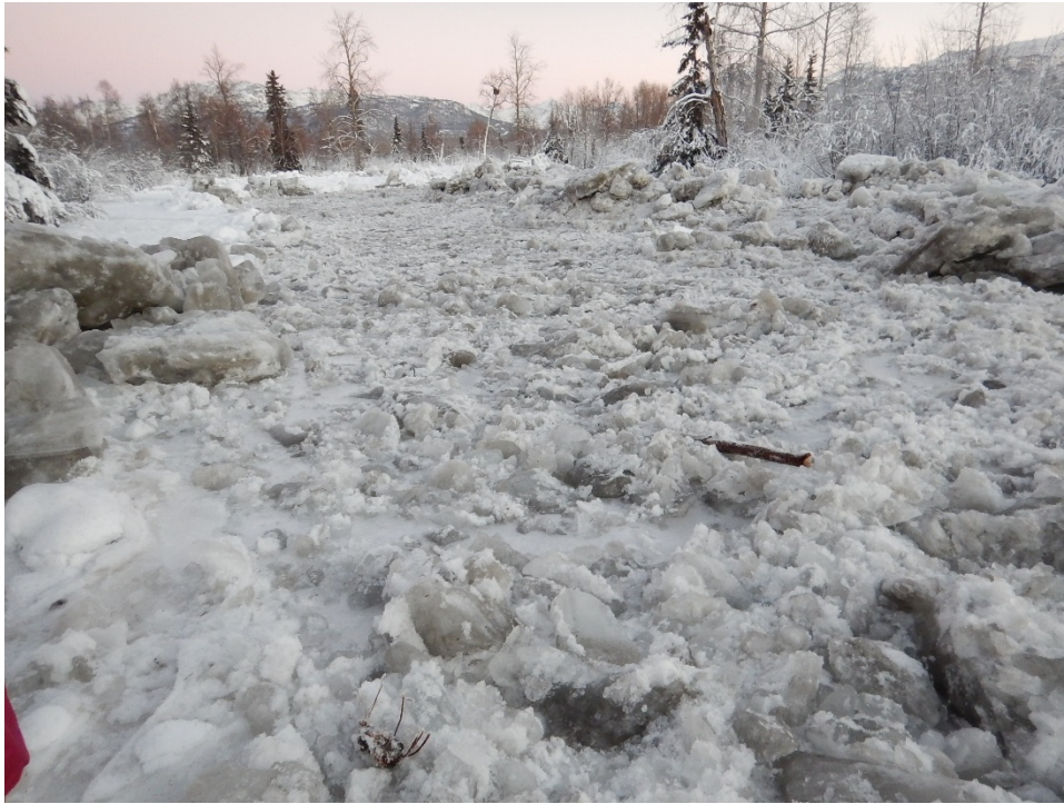
Figure 12. Ship Creek stationary ice cover after fracturing by a bulldozer.
