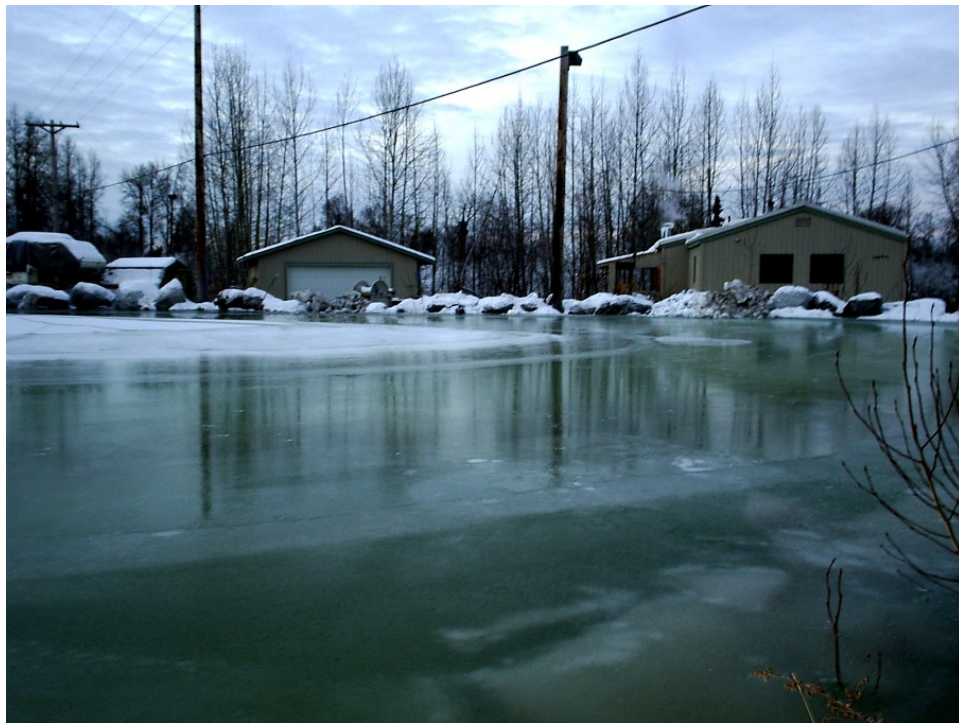
Figure 5. Inundation of buildings at the Fort Richardson Fish Hatchery. (Image by Andrea Tesch.)
