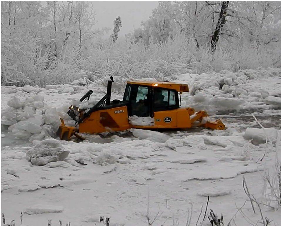
Figure 11. Breaking up the surface-ice cover (January 2017).
