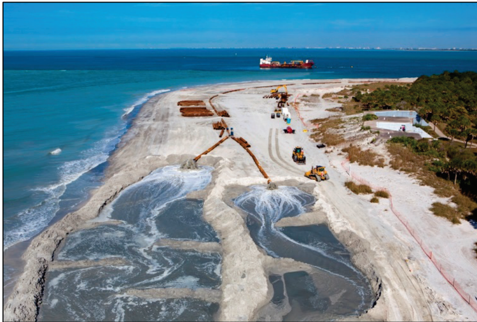
Figure 6. Traditional beach placement at northern end of Egmont Key, Florida, 26 December 2014. (Photo courtesy of GLDD.)
