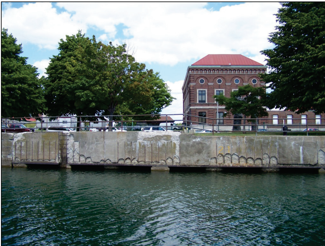
Figure 1-12. Timber pile substructure with concrete cap photograph.
