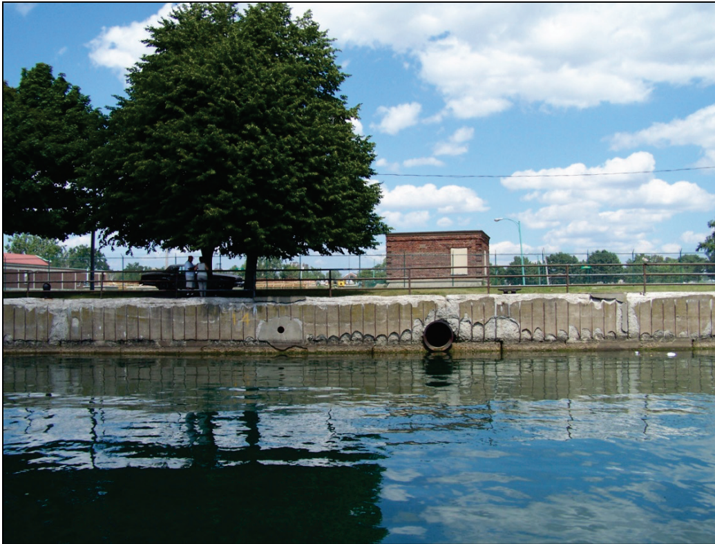
Figure 1-11. Stone-filled timber crib substructure with concrete cap photograph.
