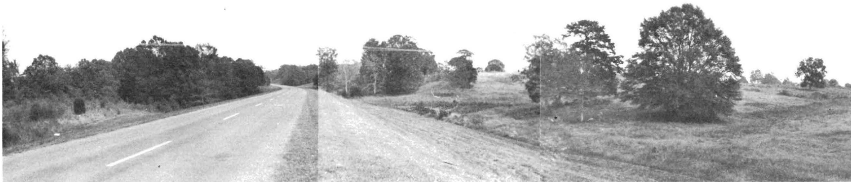
a. View northeast, road site 5
