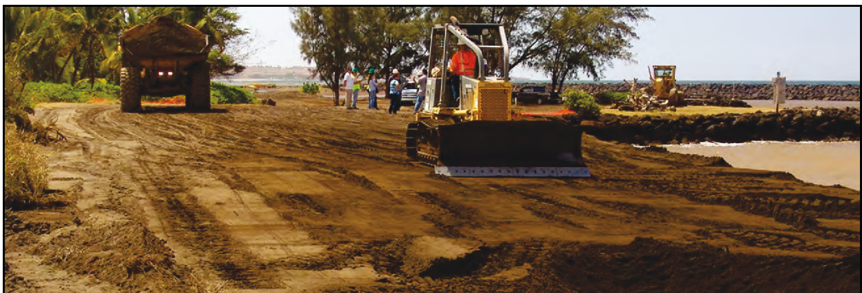
Figure 7. Placement of bypassed sand above the mean high water shoreline at the Kikiaola Harbor location during the second increment of the 2014 sand bypass operation.
