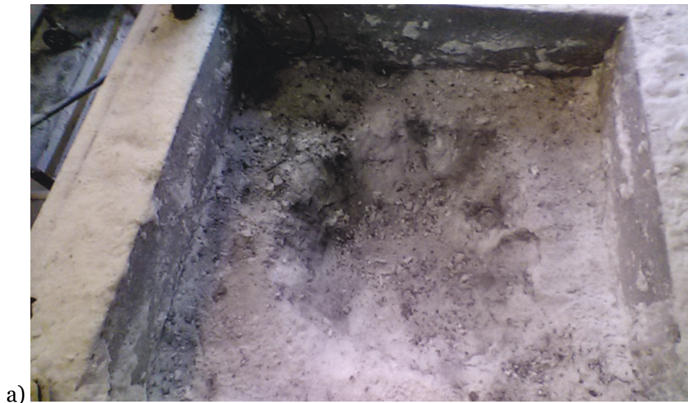
Figure 7. Fully assembled simulated crater ready for repairs with select backfill layer and capping materials: a) top view; b) side view.
