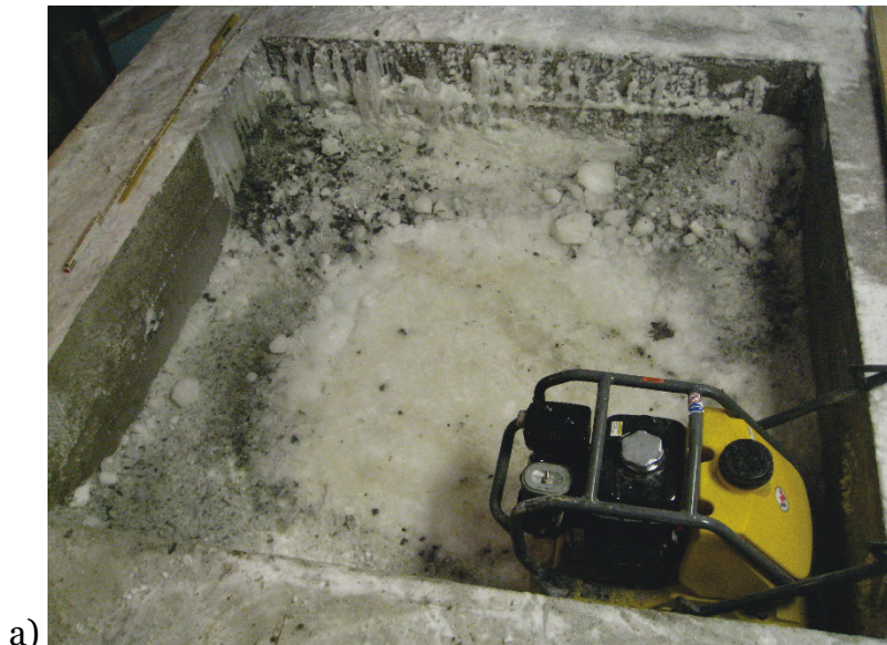
Figure 46. Repair of a full sized crater with frozen slush at -20 °F. a) The top of the backfill layer. b) Filling the cap layer with compacted frozen slush.
