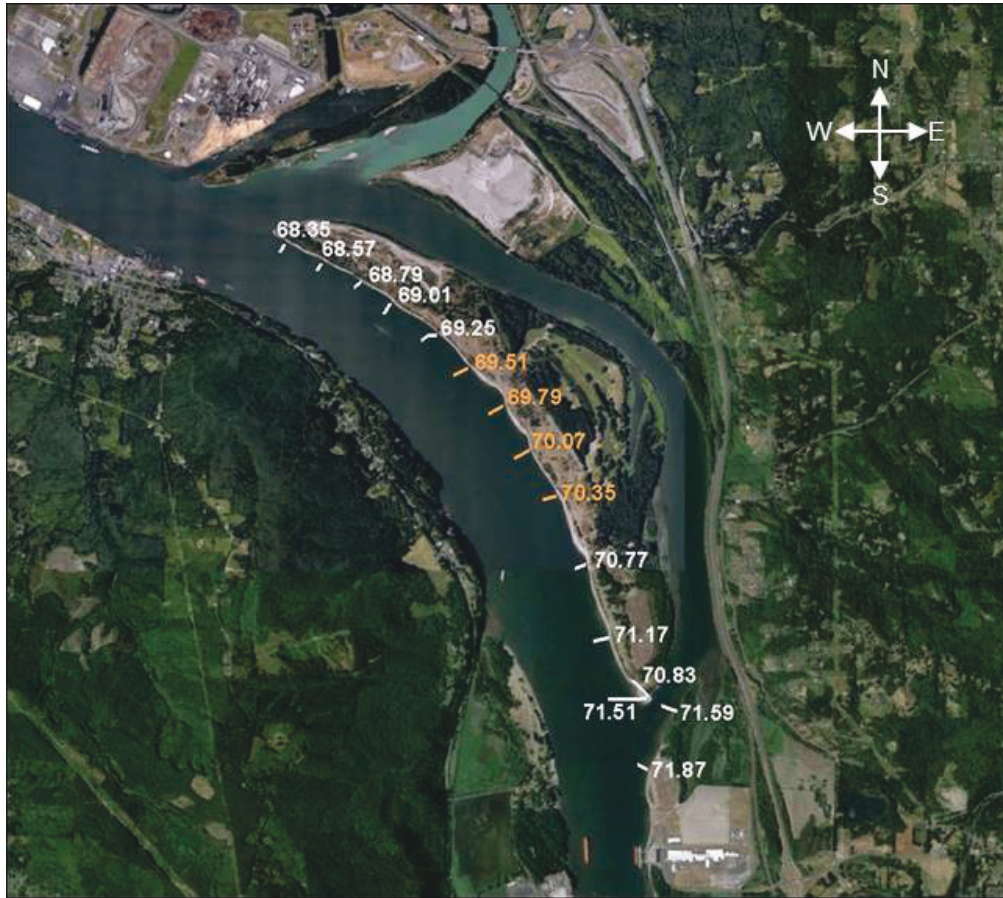
Figure 5. Dikes located to the south of Cottonwood Island.
