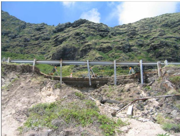
Figure 3. Erosion threatening highway along Kaupo/Kaiona beaches
