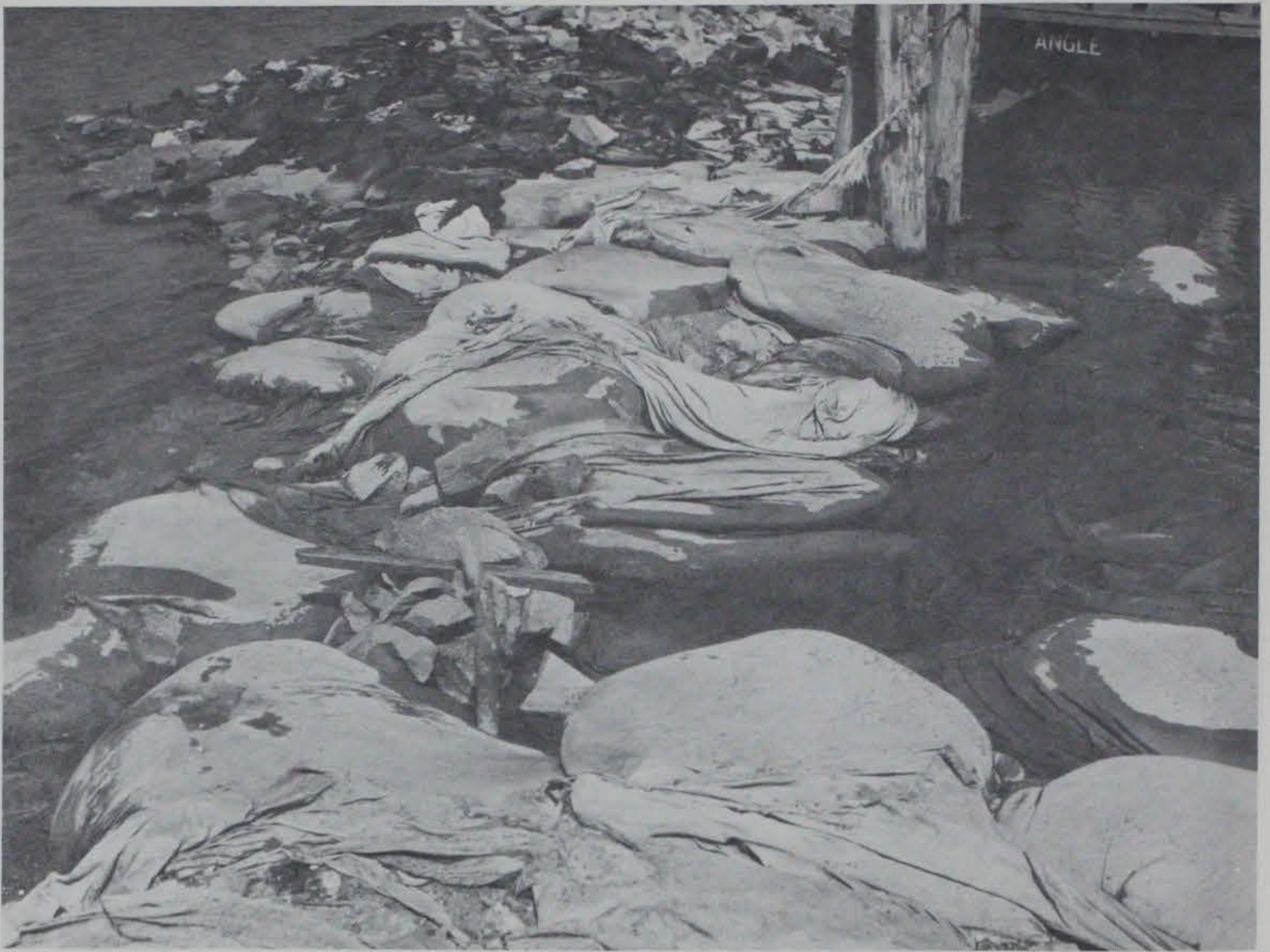
Photograph 28. Looking riverward, showing damage to both nylon and plastic bags. Note how plastic bags have shifted downstream
