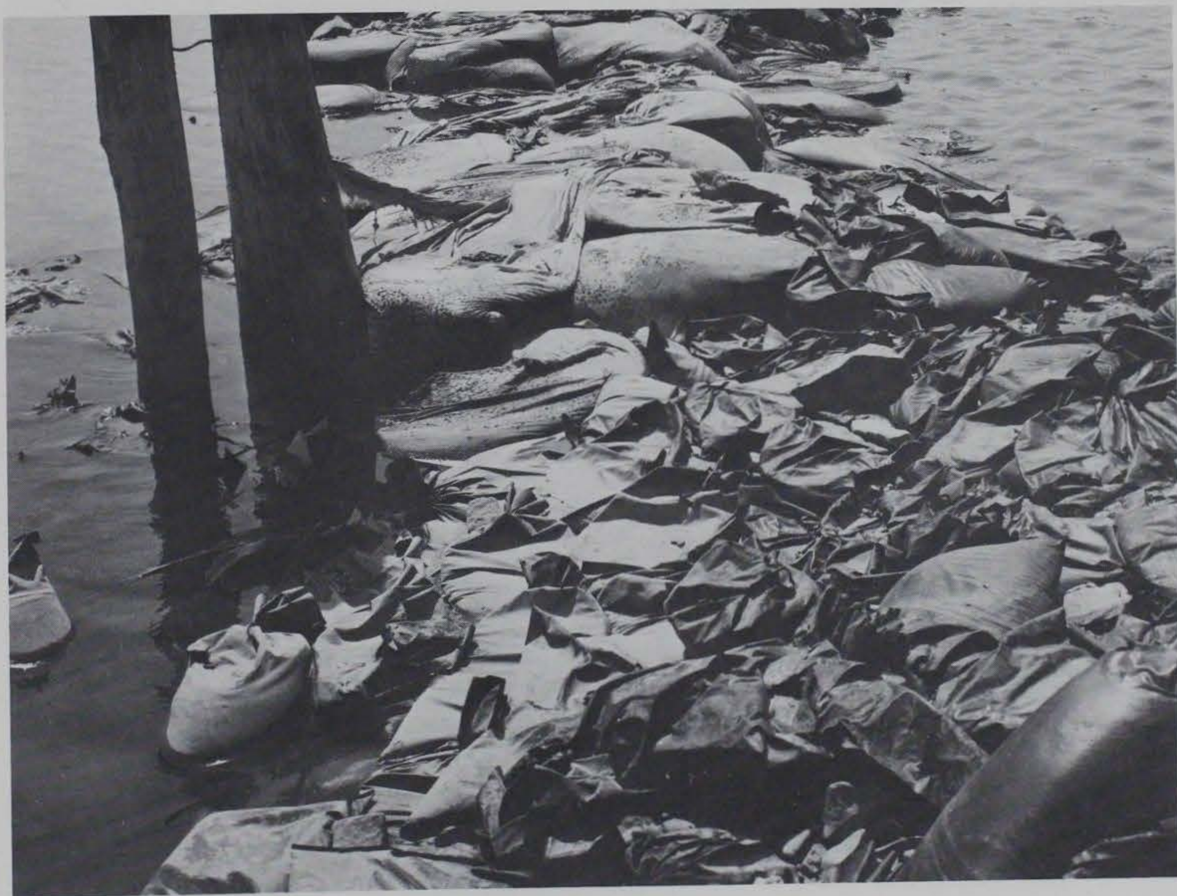
Photograph 27. Looking landward, showing damaged crown of bag dike
