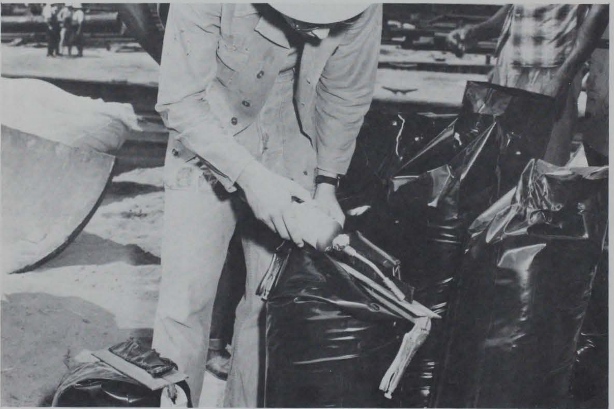
Photograph 10. Top of plastic bag being sealed by heat from a small propane torch
