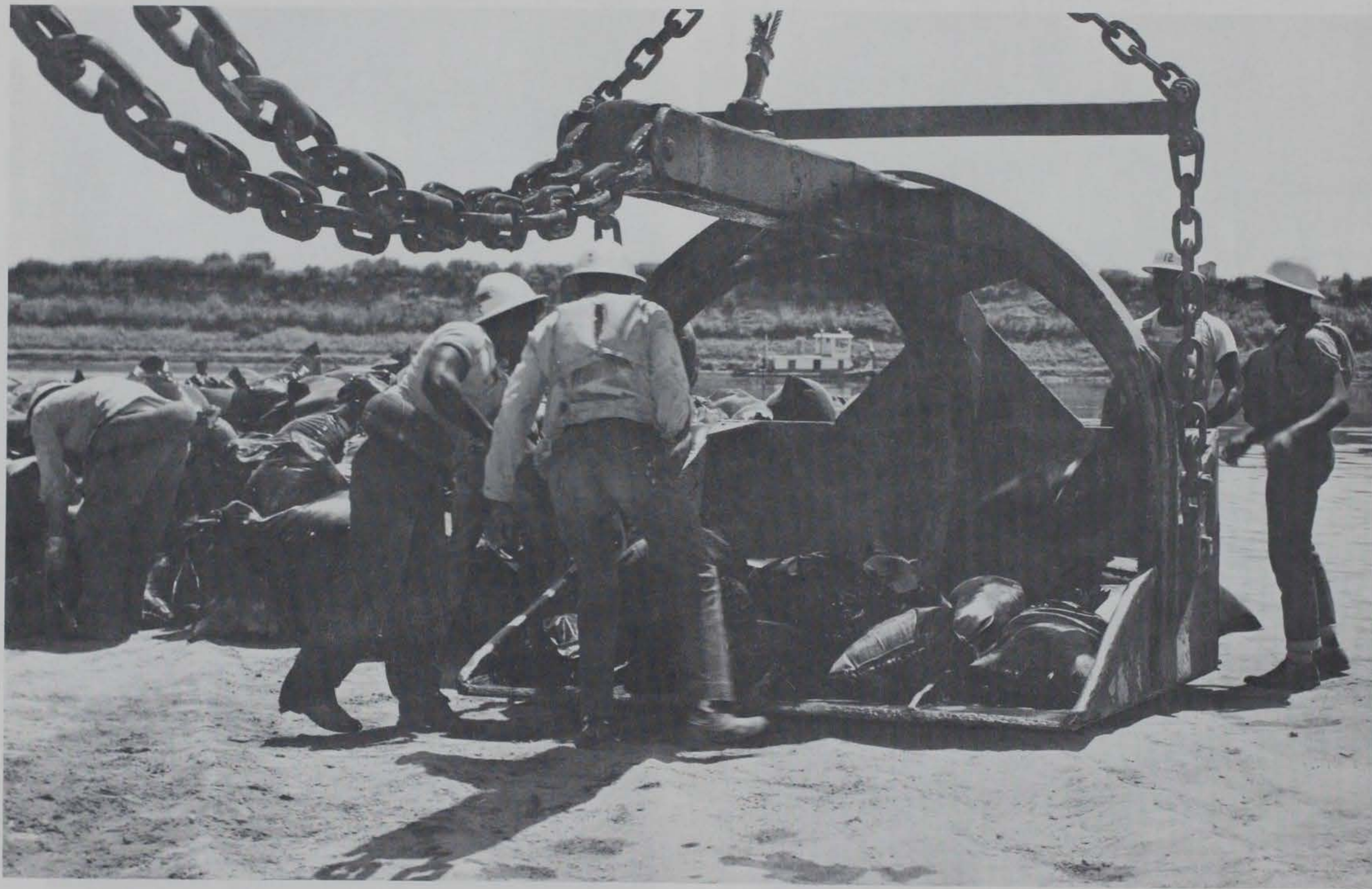
Photograph 16. Workers loading plastic bags into skip bucket
