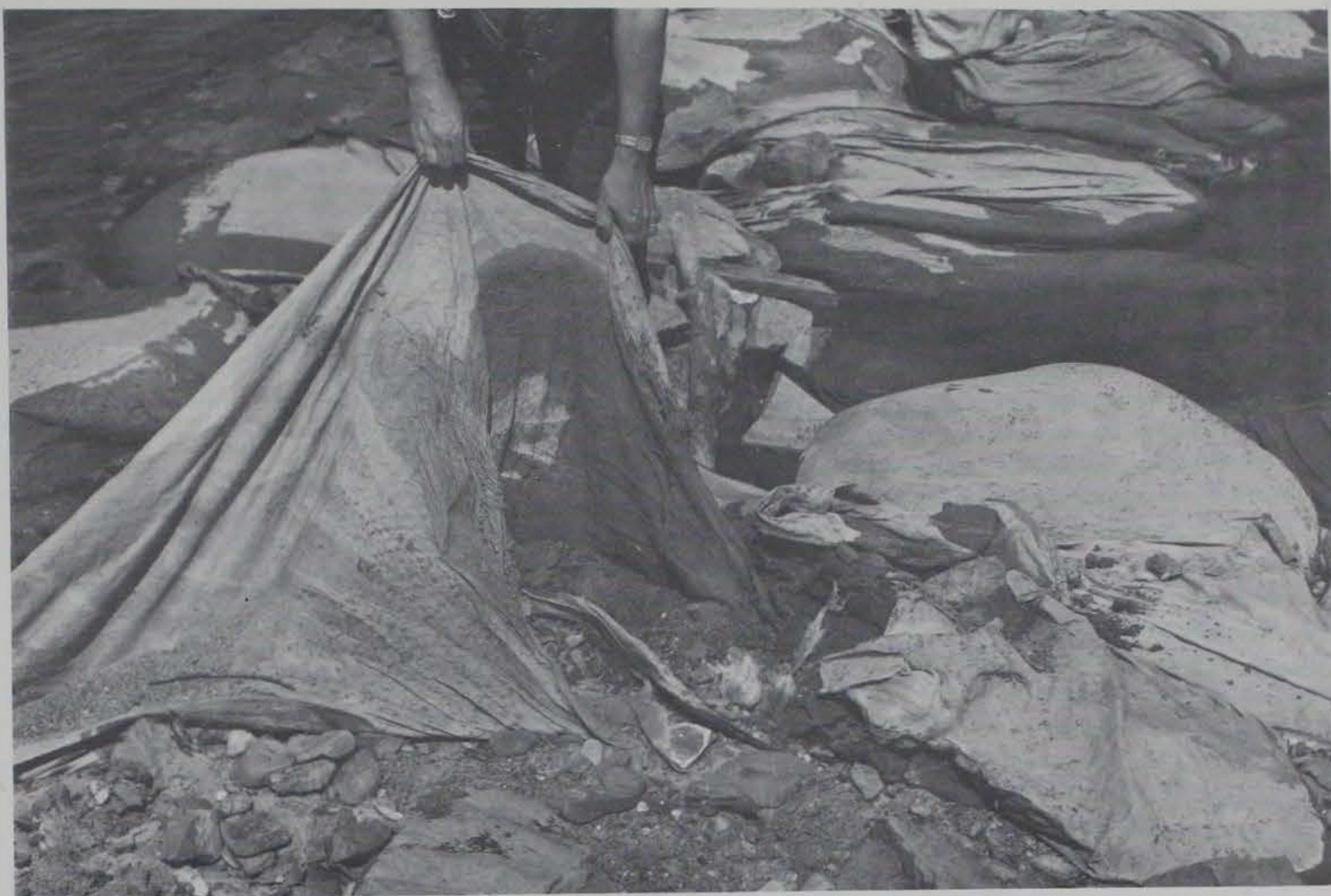
Photograph 30. Damaged nylon bags from which fill material has been lost
