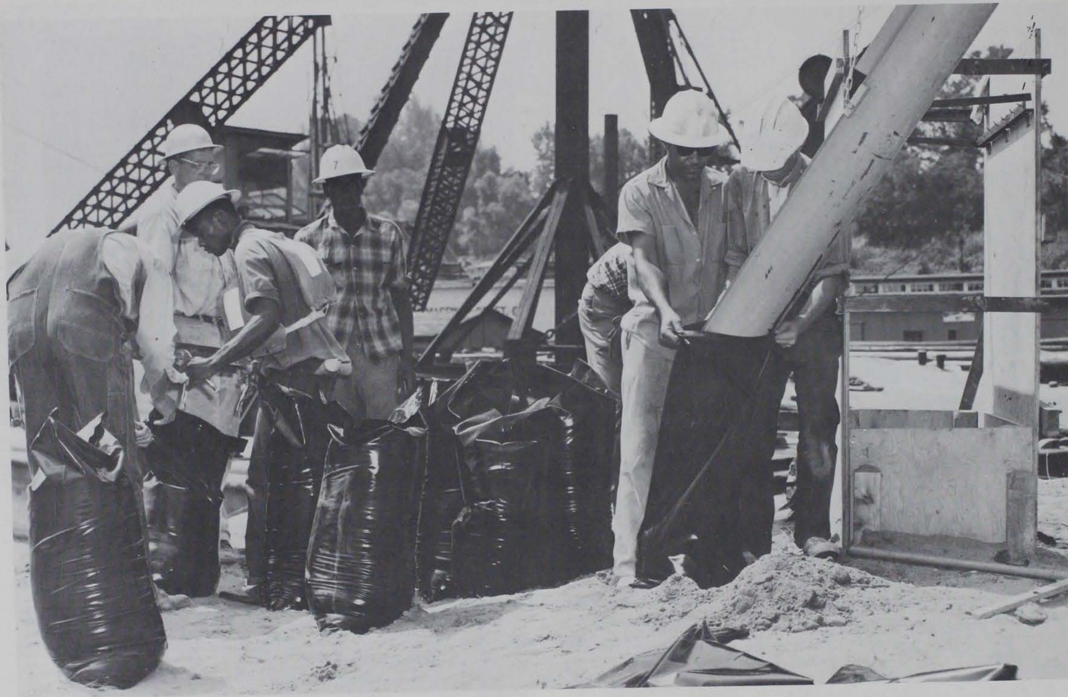
Photograph 8. Plastic bag being filled with sand from conveyor belt. Filled bags are being prepared for sealing
