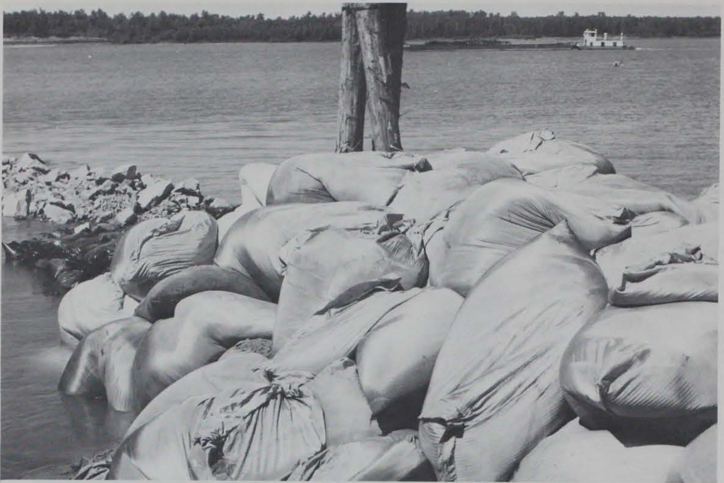
Photograph 21. Nylon bag portion complete to final grade (+8 ALWP)
