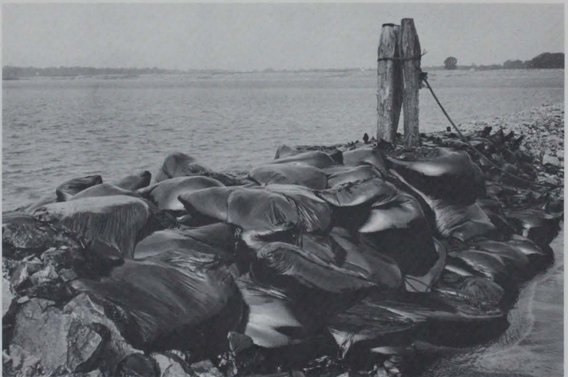
Photograph 25. Downstream views of completed nylon and plastic bag section
