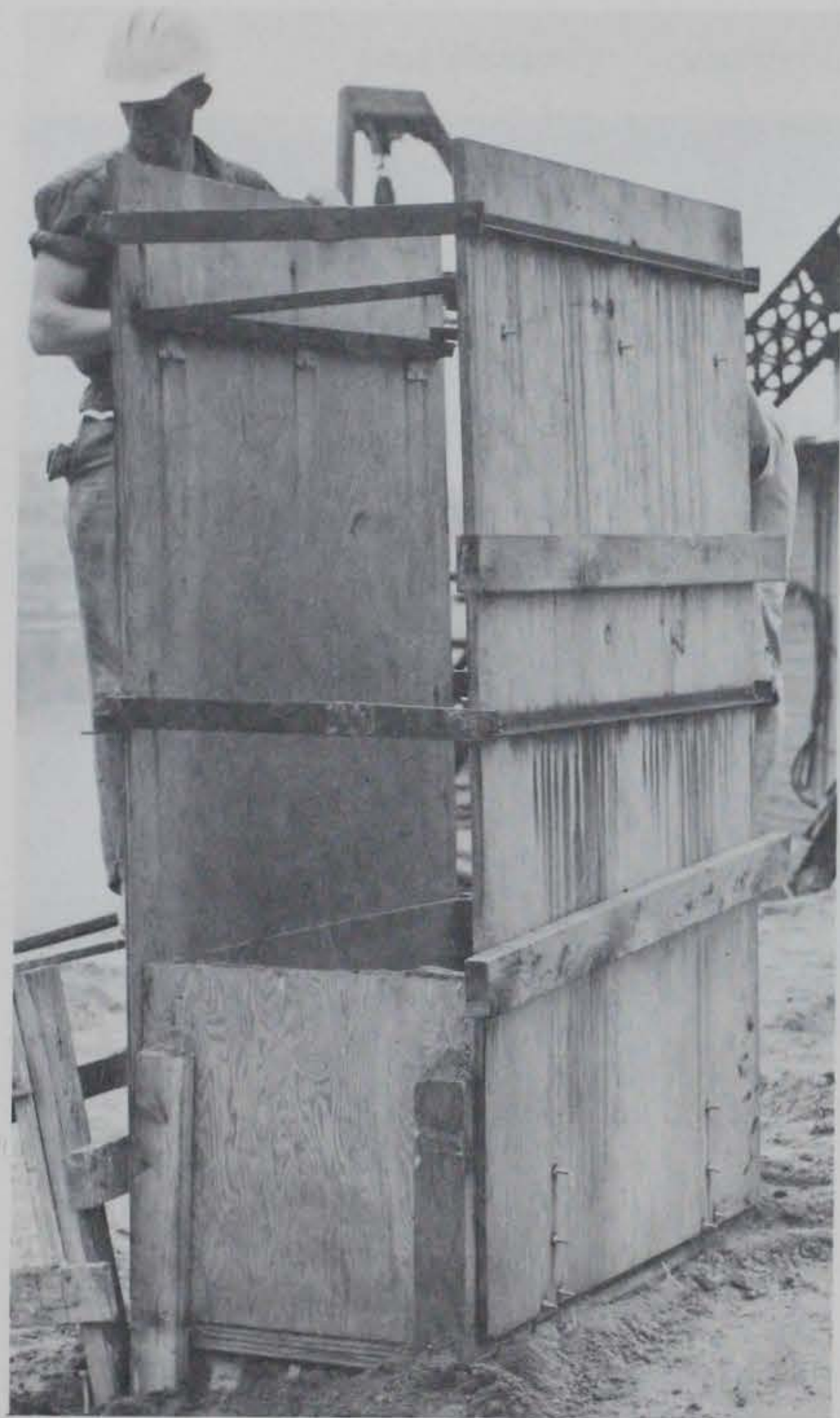
Photograph 2. Plywood box used to support nylon bags being filled with sand
