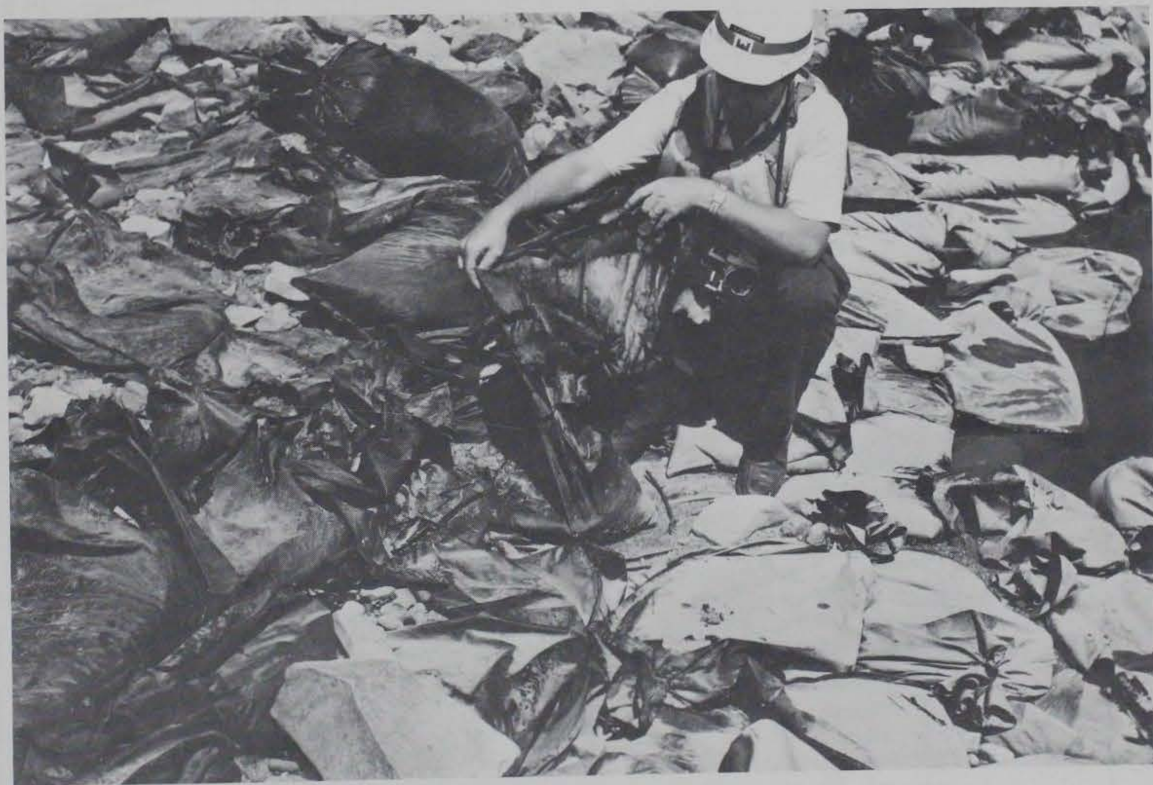
Photograph 31. Damaged plastic bags from which fill material has been lost
