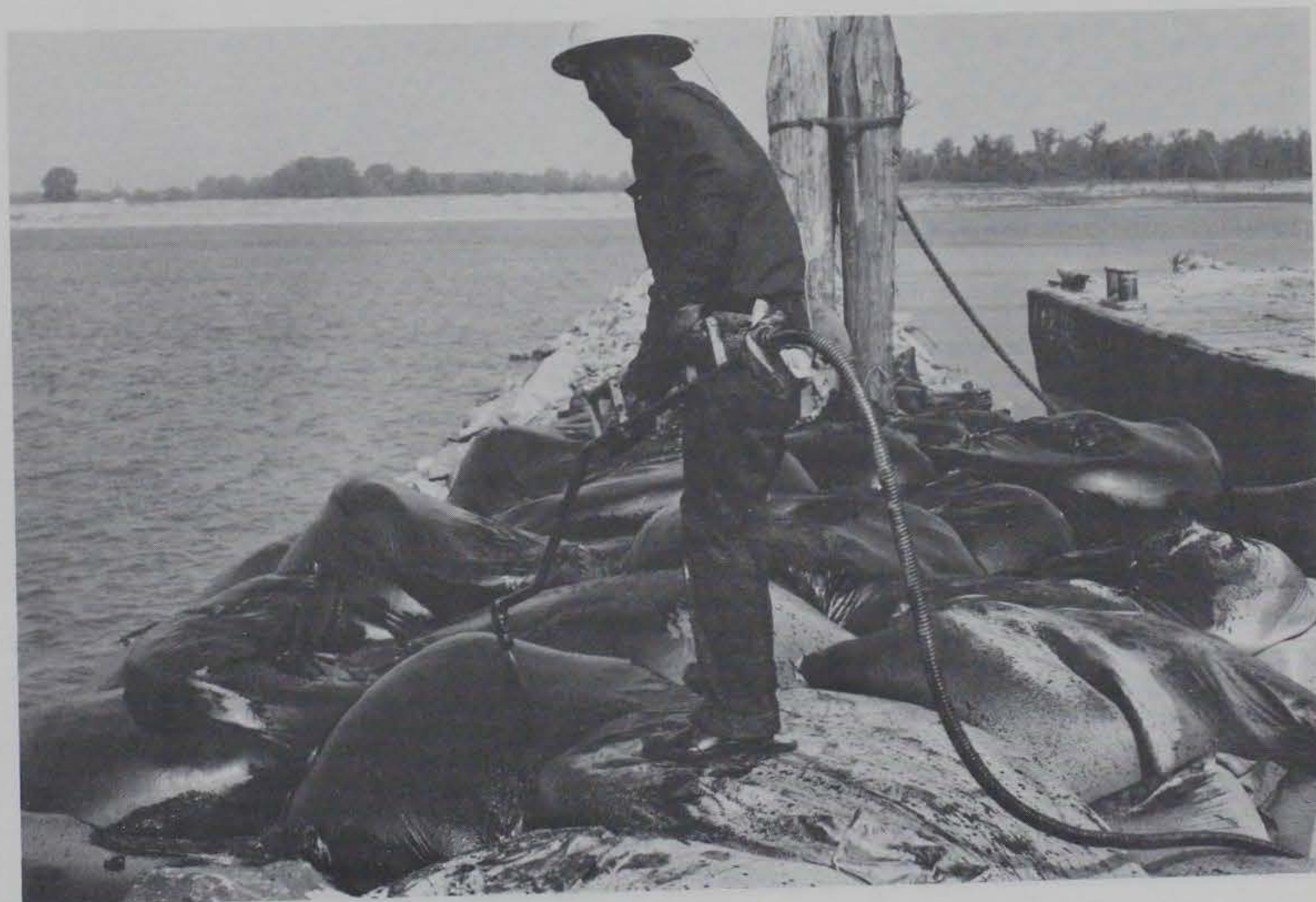
Photograph 24. Spraying nylon bags with coal-tar emulsion
