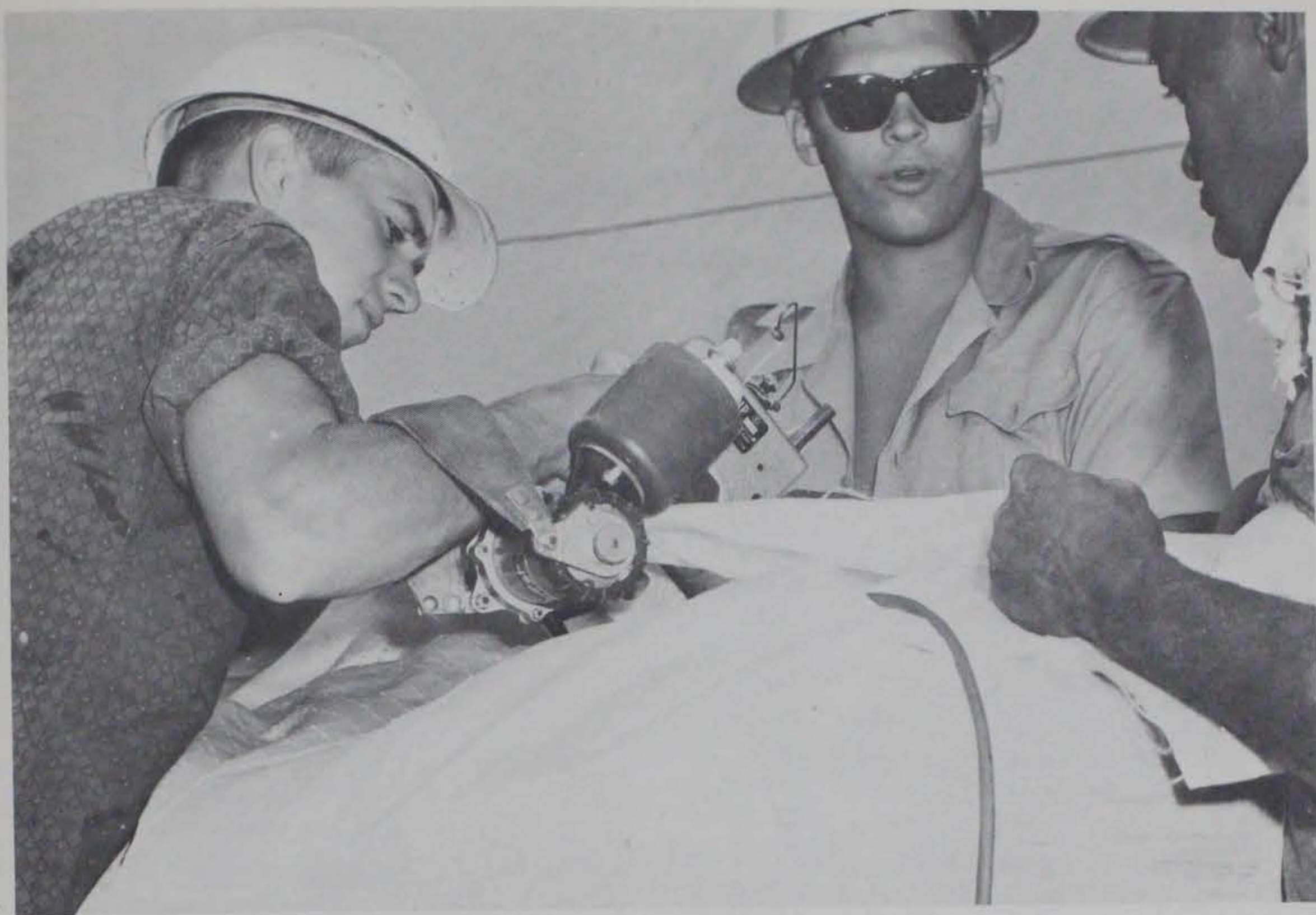
Photograph 4. Sewing nylon bag with special portable sewing machine
