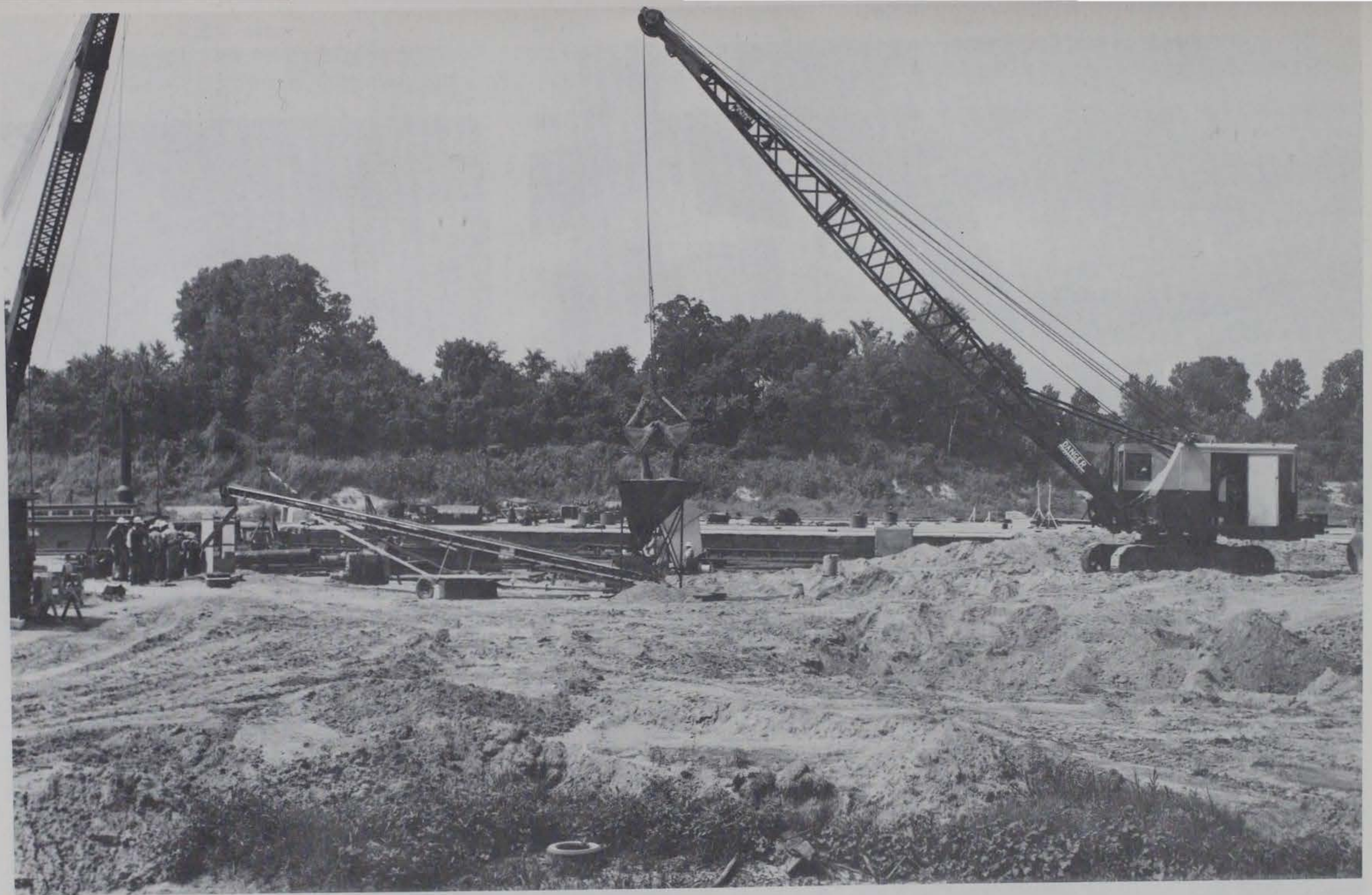
Photograph 1. Overall view of borrow area showing equipment used in filling nylon and plastic bags
