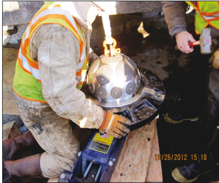
Figure 14. A self-lubricating pintle bearing.
