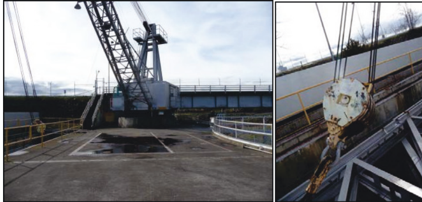
Figure 27. Large crane and hoist at the John Day Dam.
