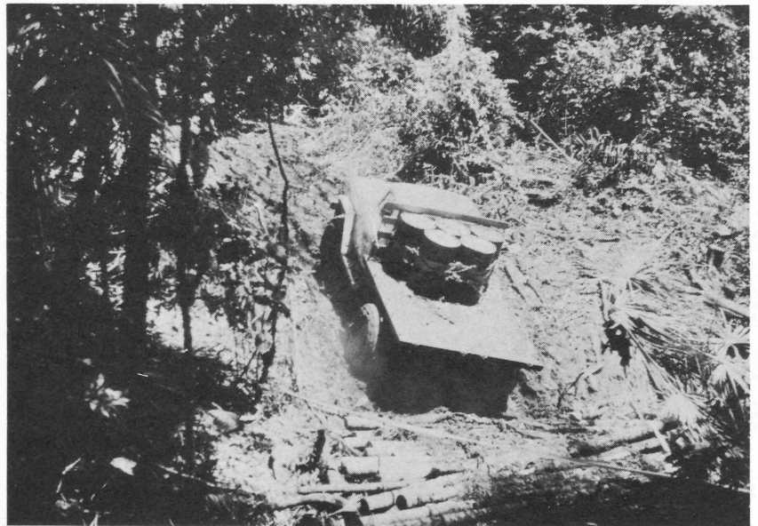
Fig. 7. Power wagon crossing a stream on crib-bridging, Swamp Fox II
